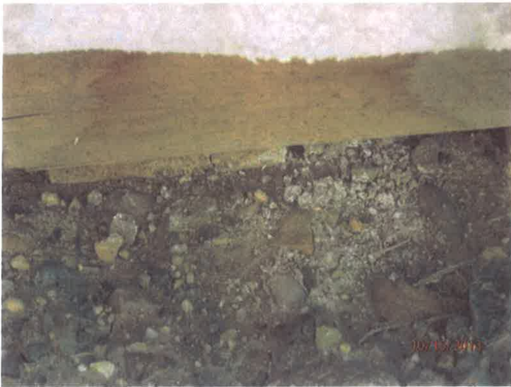
Photo 8 Third container (alternate view) - leached waste through container liner onto soil.
