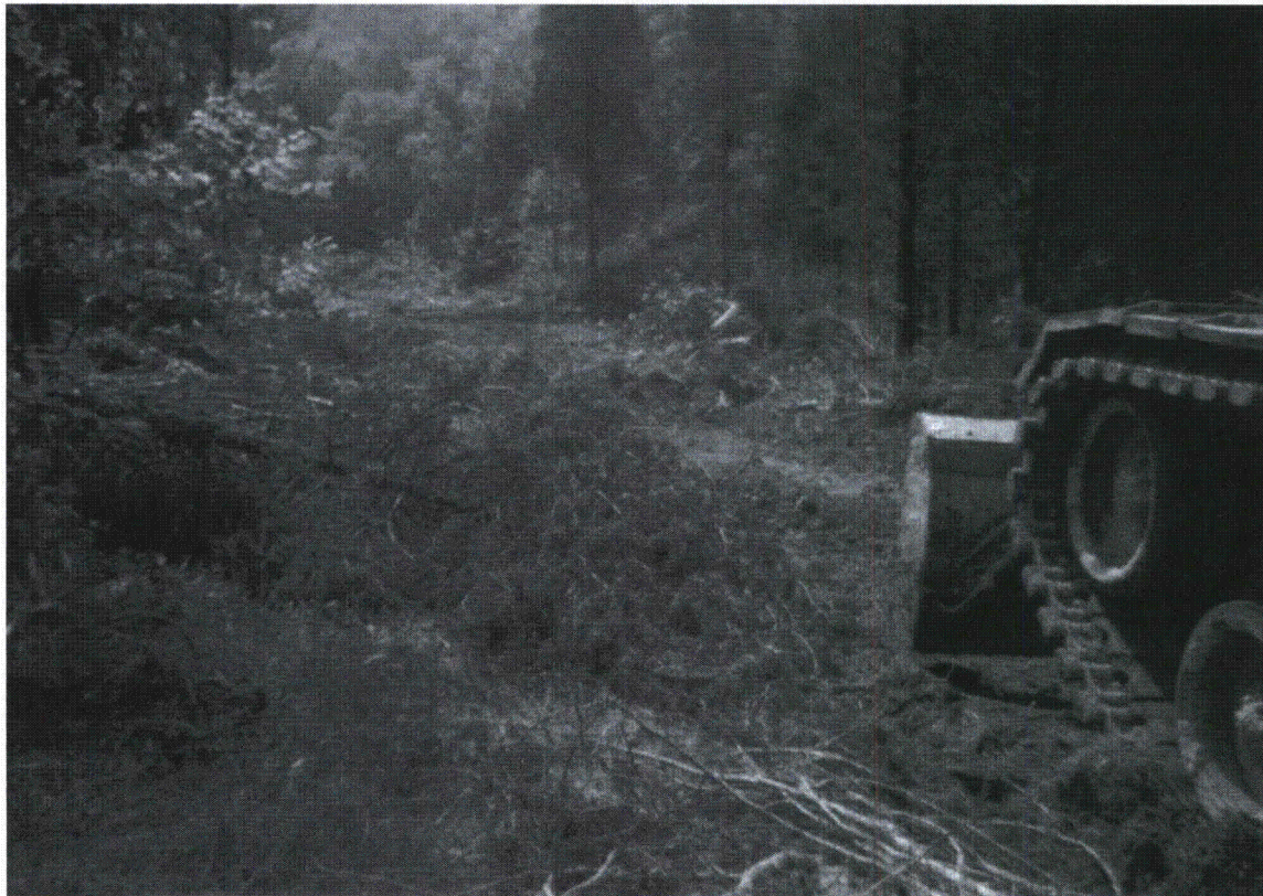
Armored dozer used by Larry to create line of sight for surveyors on Emergency Landing Road.
