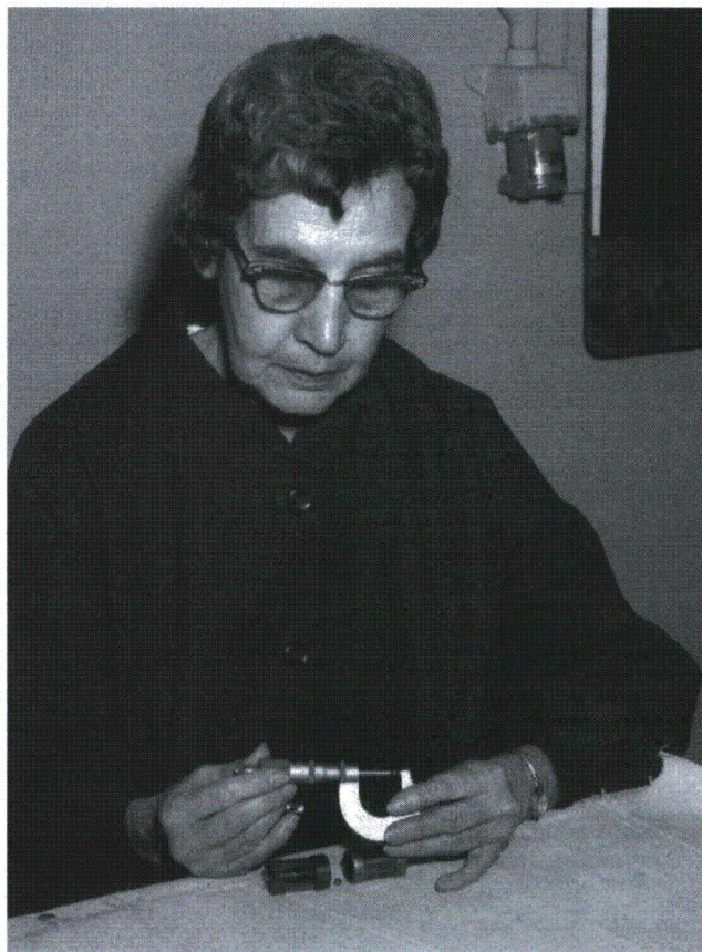
Nellie Jones measuring the width of copper crushers to obtain chamber pressure after firing.
