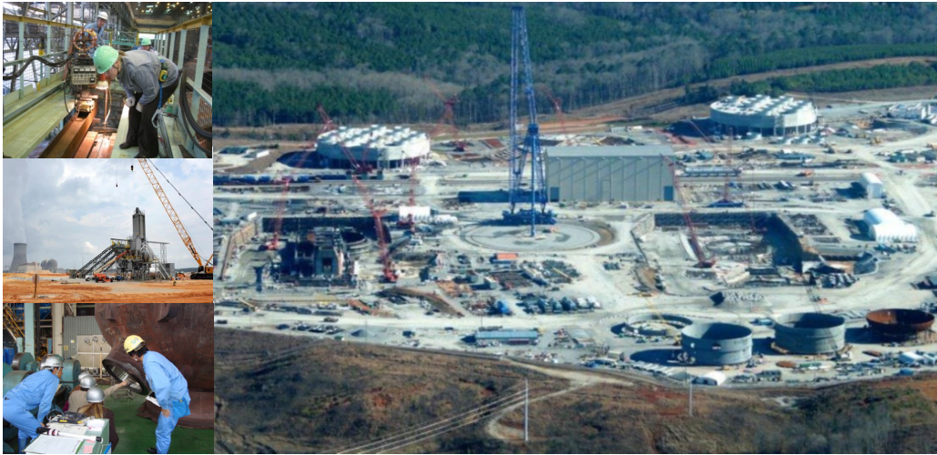
VC Summers 2 & 3 – Construction Site 2014
