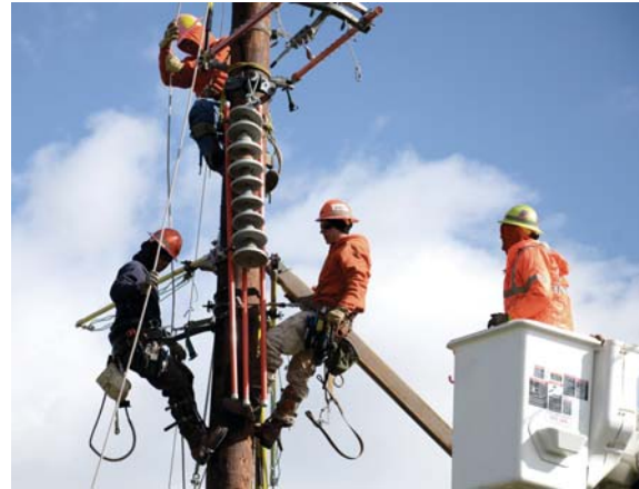
// Forward Progress: Candidates for electric lineman apprentice positions participate in exercises at the new Metro East Training Center in Belleville, Ill., where workers are learning about the latest "smart" technologies for electric and gas delivery service. The facility opened in October 2013 as part of Ameren Illinois' Modernization Action Plan to create jobs and enable energy innovation.
