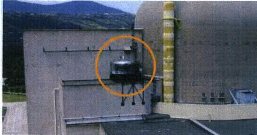
Figure A1.2: picture of the sand bed filter as implemented in the PWR 1300 MWe of Nogent sur Seine
