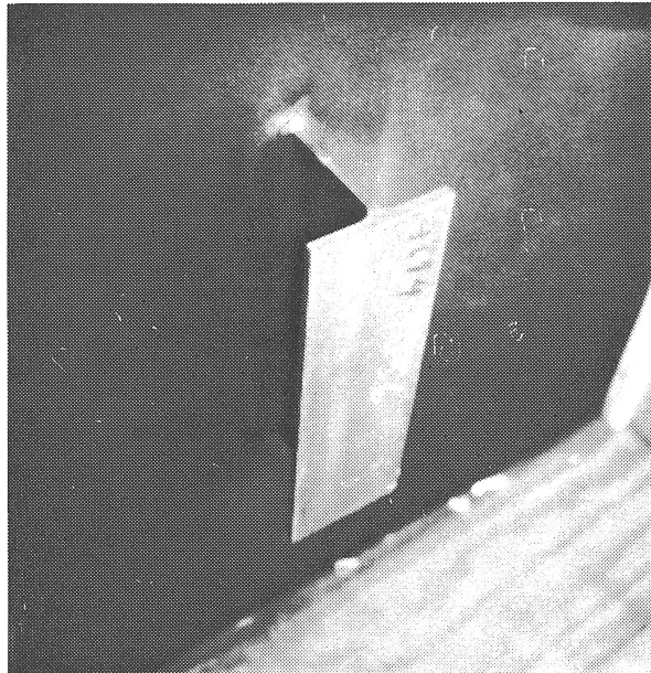
Plate 1: Close-up of tee welded to liner plate
