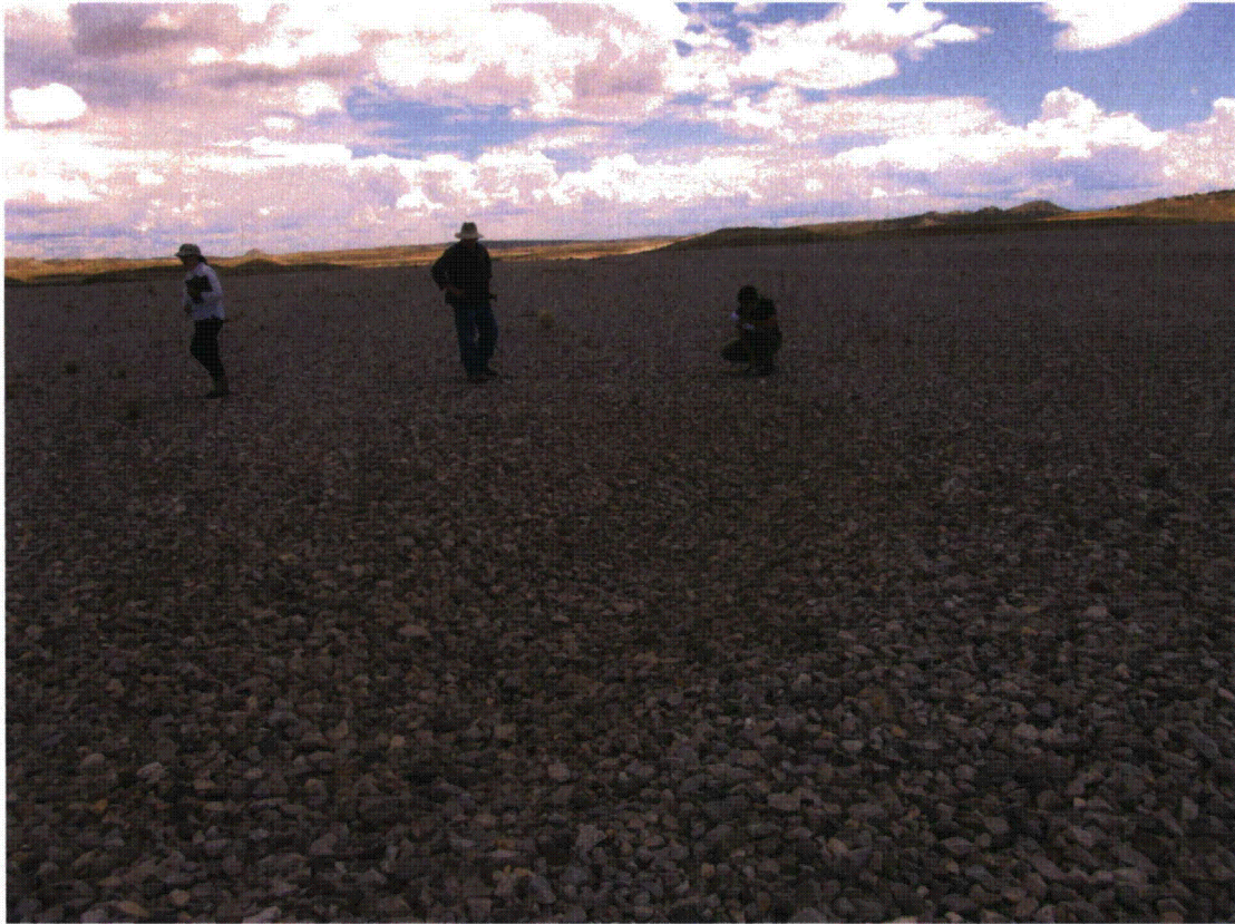
MAW 8/2014. PL-7. Shallow depression on top of disposal cell.
