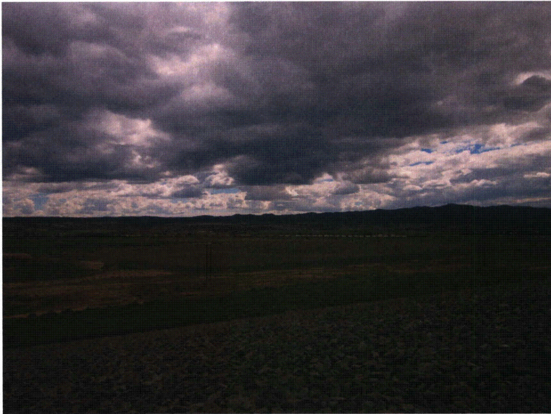
BLU 8/2014. PL-9. Carbonate tailings disposal cell viewed from main tailings disposal cell.
