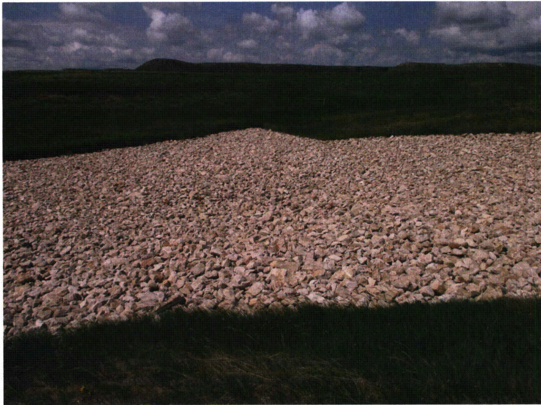
EDG 7/2014. PL-7. West diversion channel.
