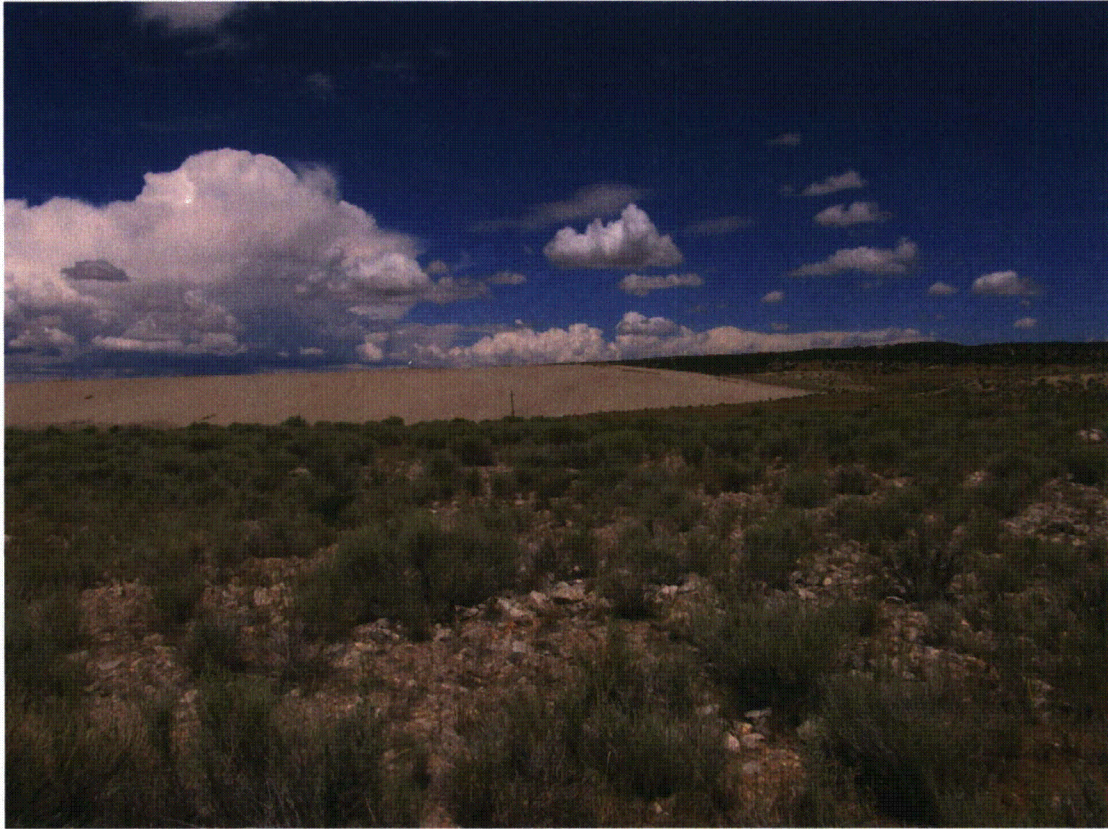
MAW 8/2014. PL-3. Southeast portion of disposal cell.
