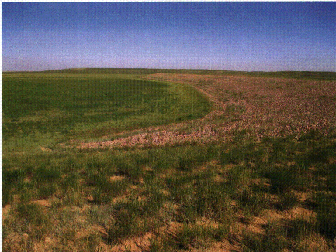
SBS 7/2014. PL-6. Riprap-armored slope between disposal cell upper and lower surfaces.
