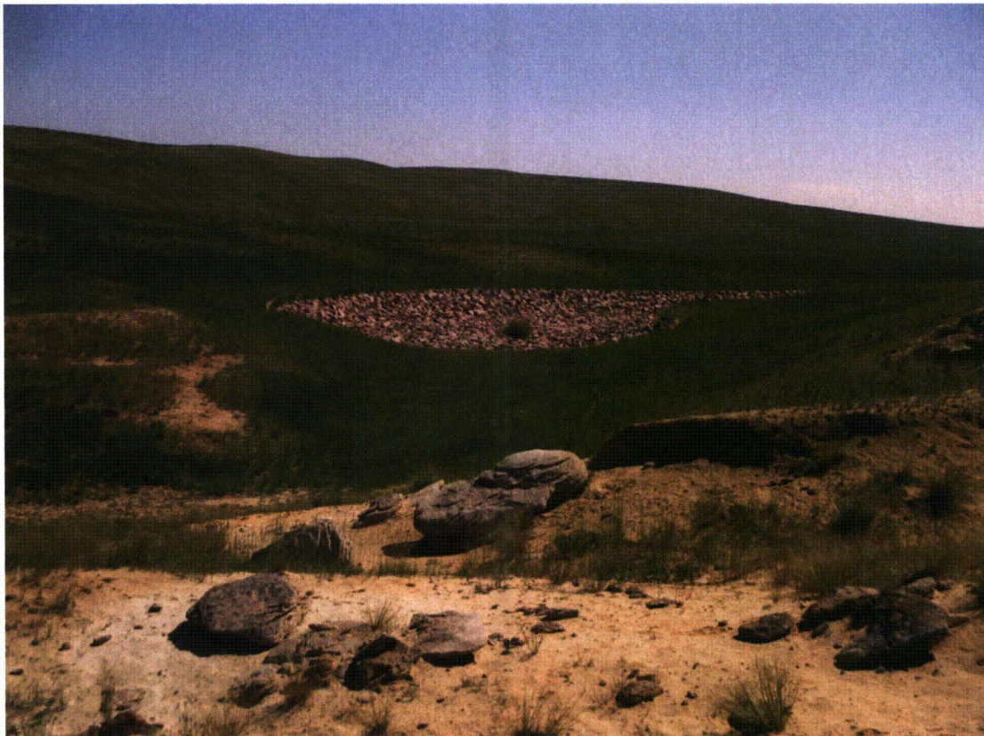
SBS 7/2014. PL-8. Outlet of riprap-armored drainage channel.
