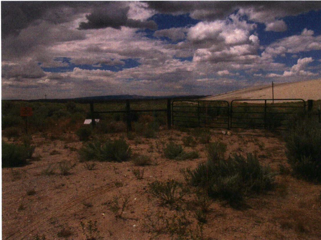
MAW 8/2014. PL-1. Entrance gate, entrance sign, and site marker (disposal cell in background).
