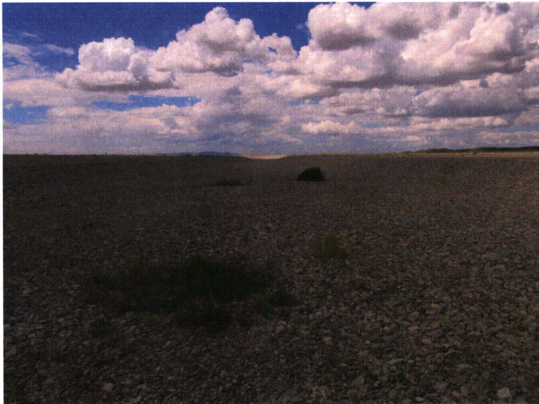
MAW 8/2014. PL-5. Diversion Channel No. 1 on top of disposal cell.
