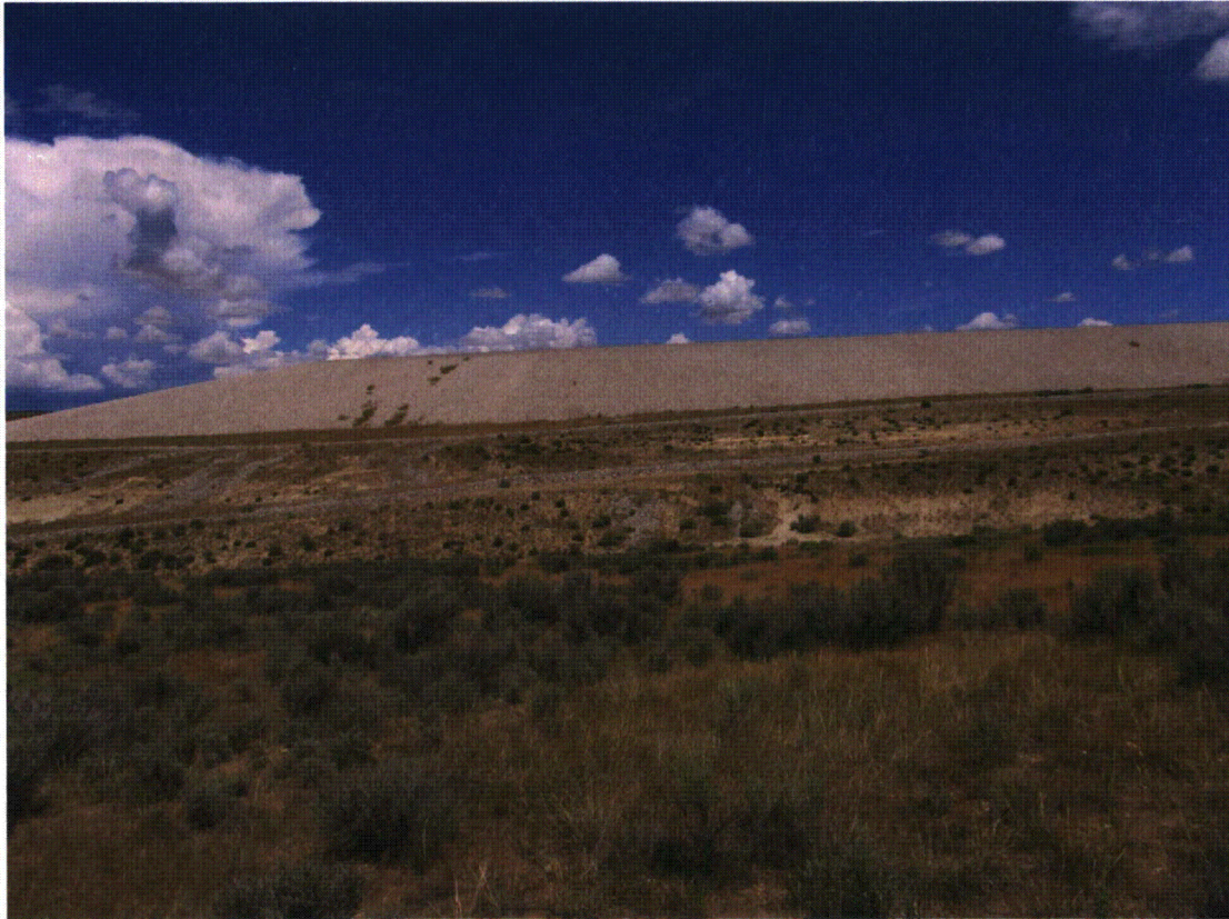
MAW 8/2014. PL-11. Diversion Channel No. 2 (rock berms and southwest portion of disposal cell in background).
