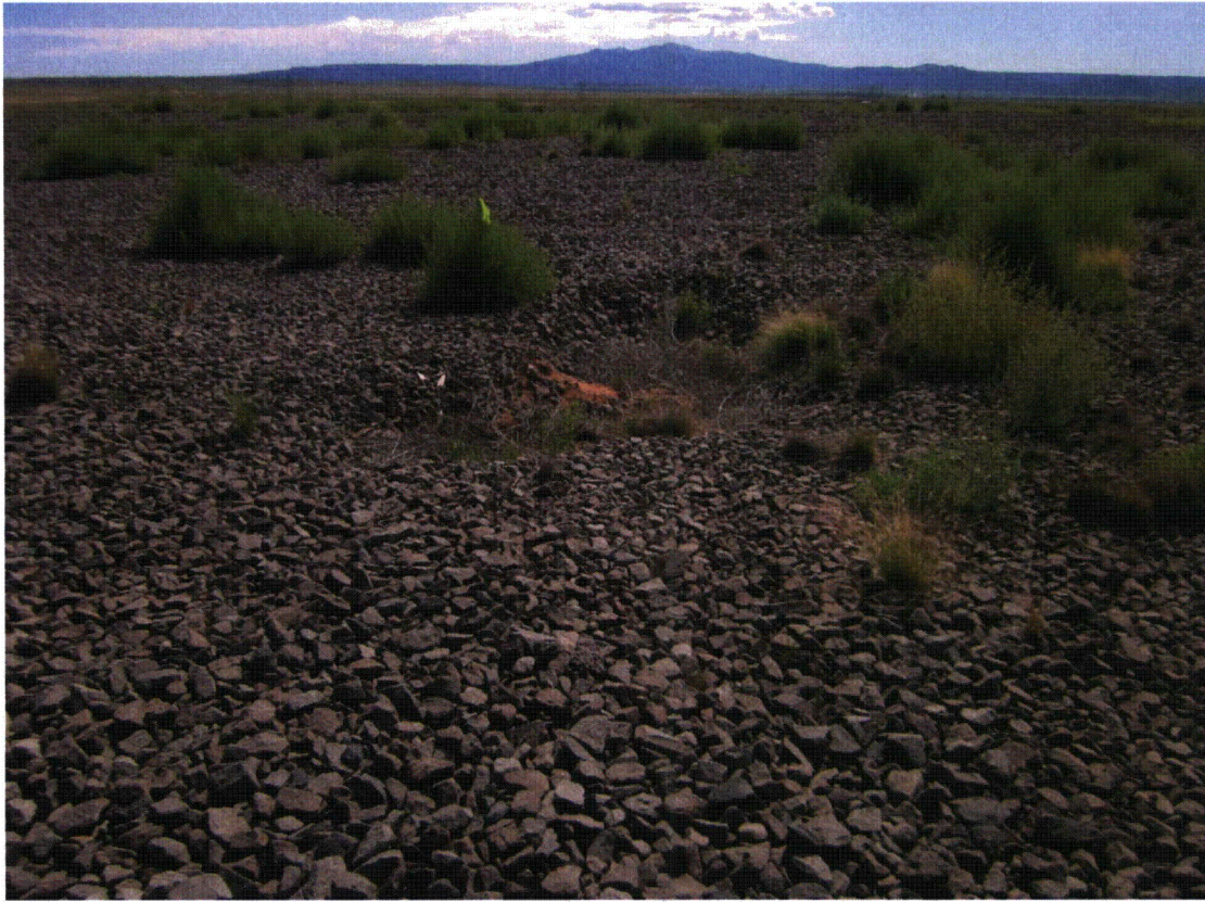
BLU 8/2014. PL-11. Depression on top slope of carbonate disposal cell.
