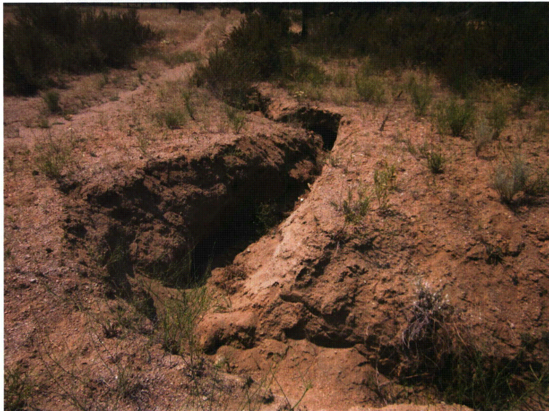
SHE 7/2014. PL-4. Erosion near perimeter sign P2.
