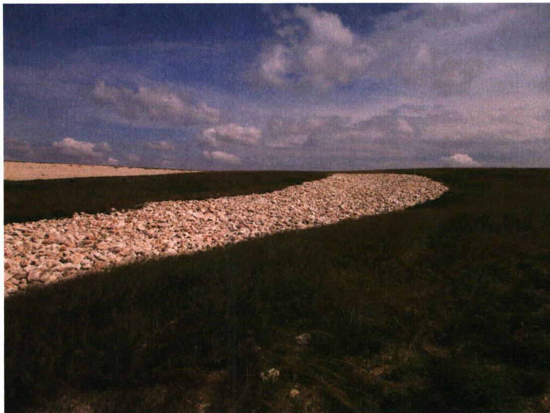
EDG 7/2014. PL-6. East diversion channel.
