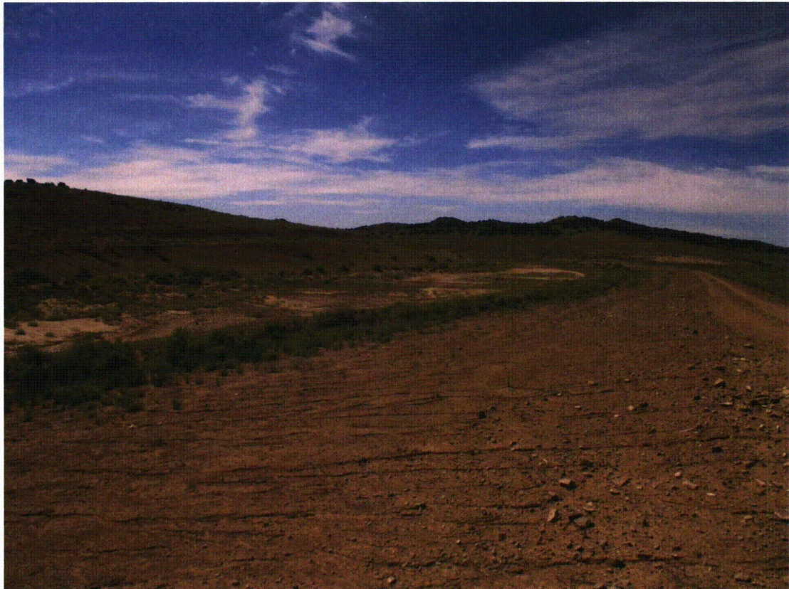
BAR 8/2014. PL-8. East diversion channel.
