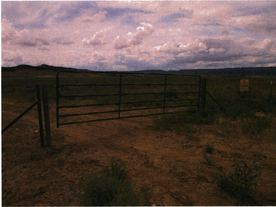
BAR 8/2014. PL-3. Site entrance gate.
