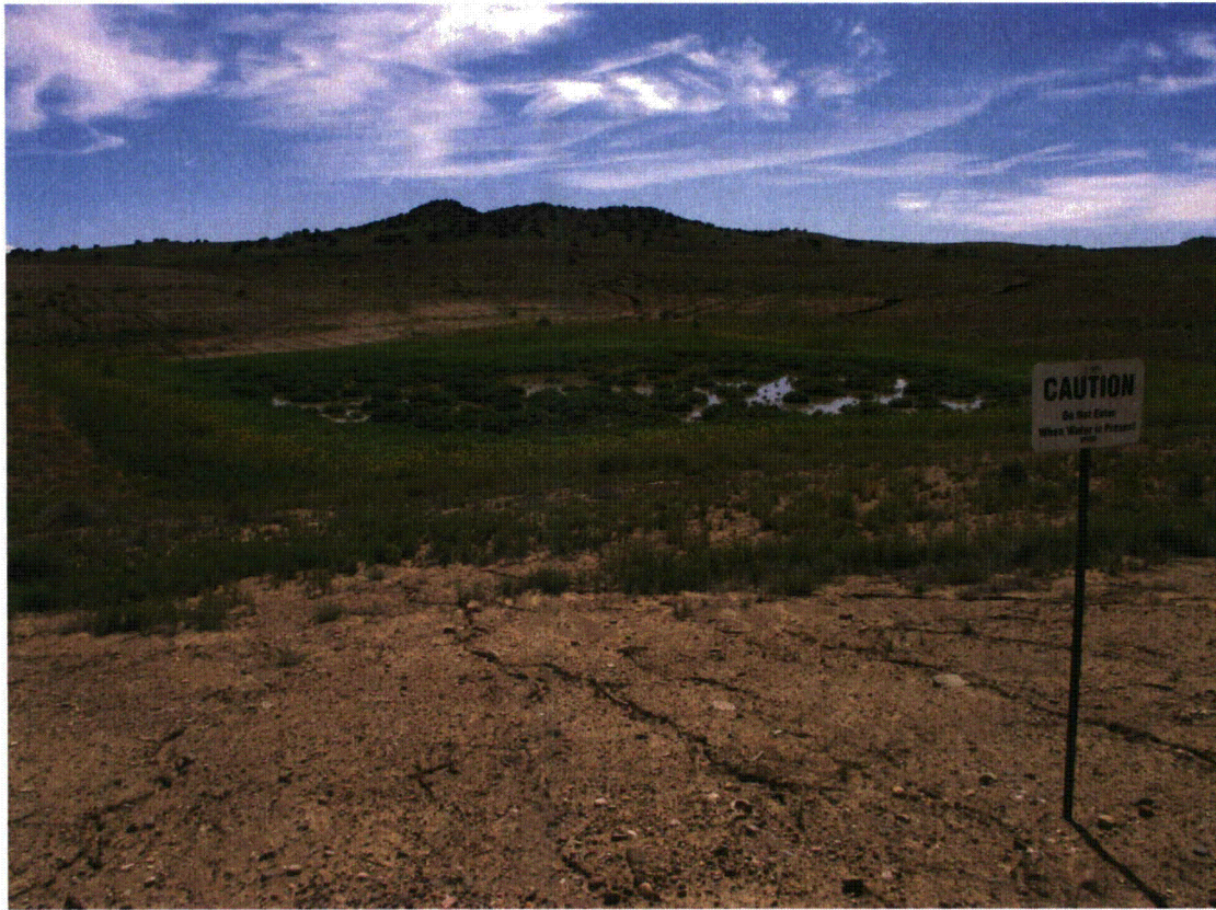
BAR 8/2014. PL-9. Vegetation and standing water in sediment trap.
