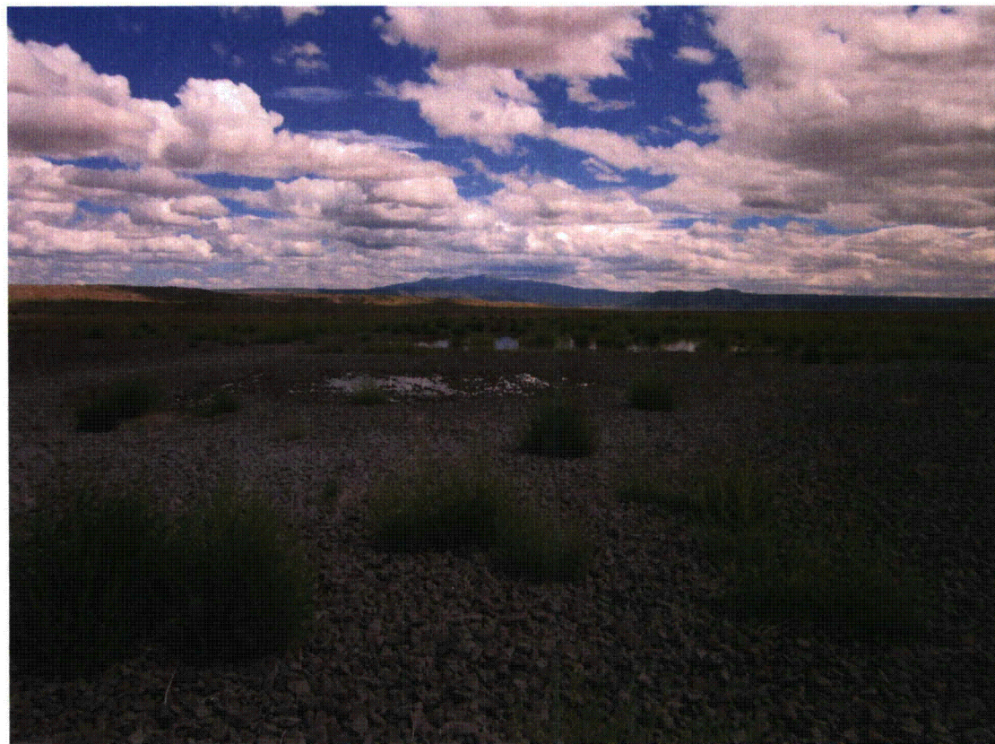
BLU 8/2014. PL-8. Ponded water in shallow depressions on main tailings disposal cell top slope.
