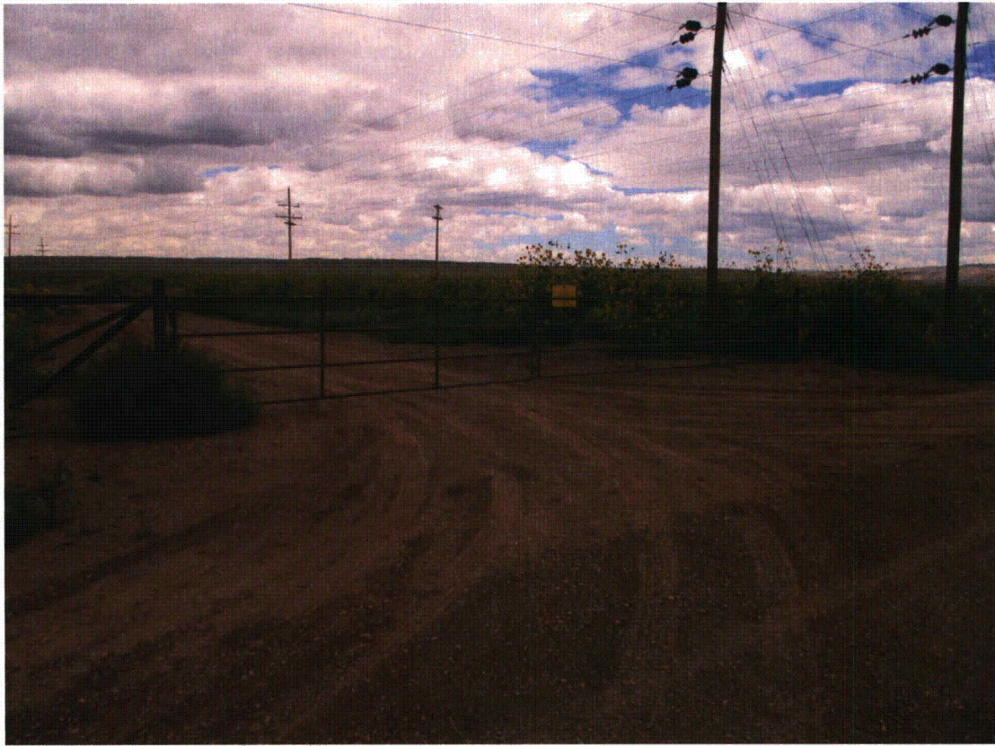
BLU 8/2014. PL-1. Site entrance gate.
