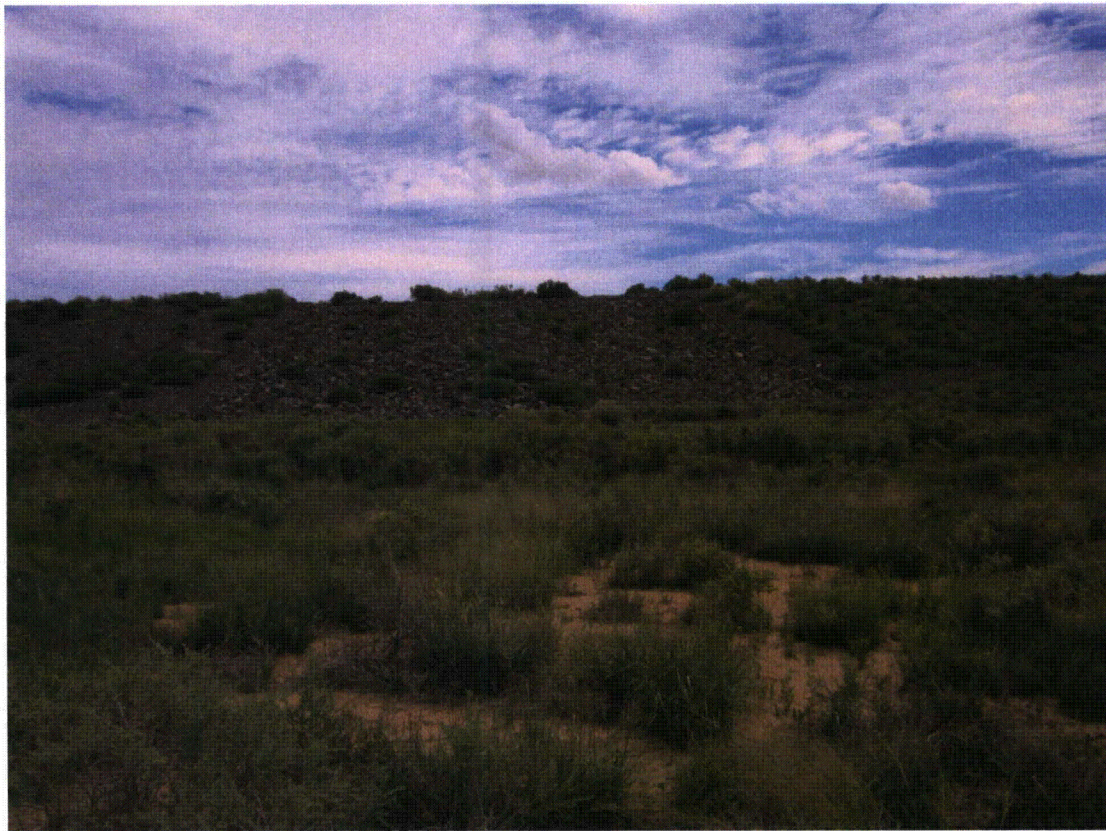
BAR 8/2014. PL-6. Rock-armored tailings impoundment spillway.
