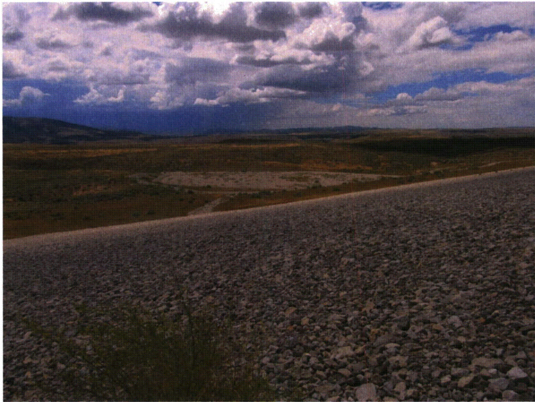
MAW 8/2014. PL-9. South side slope of disposal cell (ancillary cell in the background).
