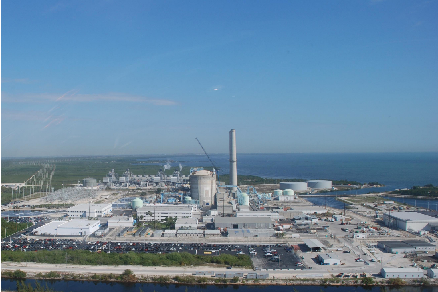
Figure 3.1-1 Existing Turkey Point Units 1 to 5
