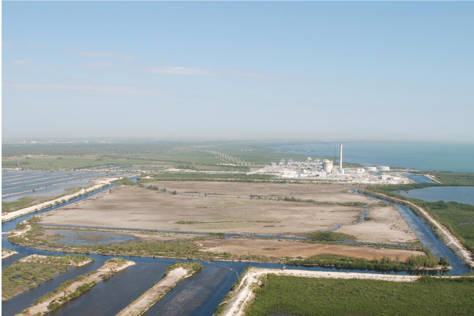
Figure 3.1-2 View of Location of Units 6 & 7 with Existing Units 1 to 5 in Background
