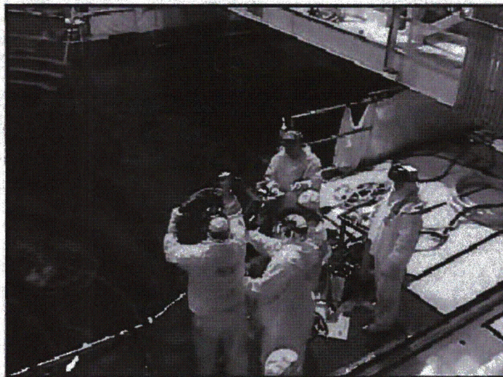
Figure 3. Typical AIRIS 21 Removal from an RPV Cavity
