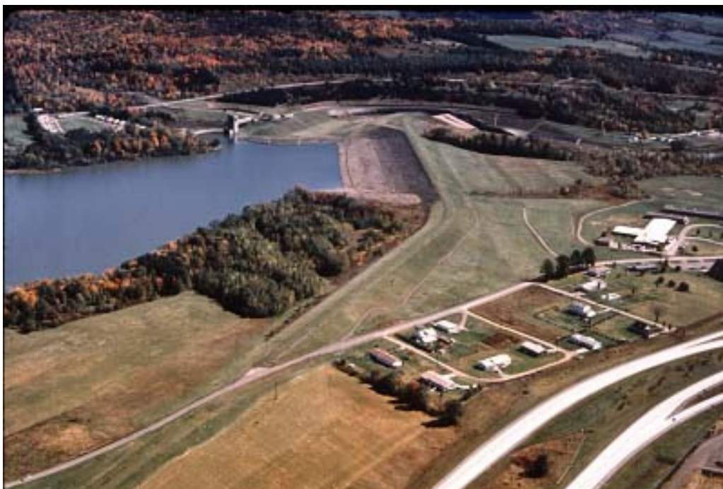
Figure 12. Photo of Whitney Point Dam, forming Whitney Point Lake
