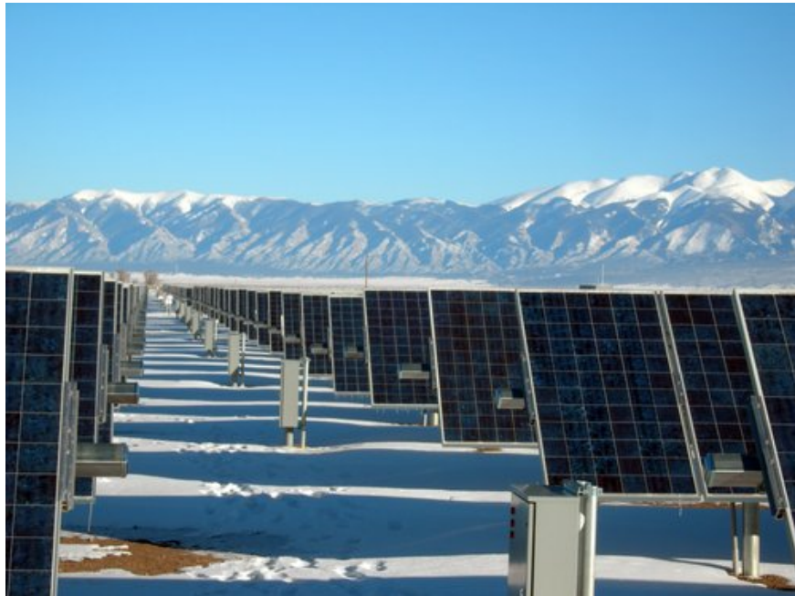
Figure 14. SunEdison's 8.2 MW Alamosa plant
