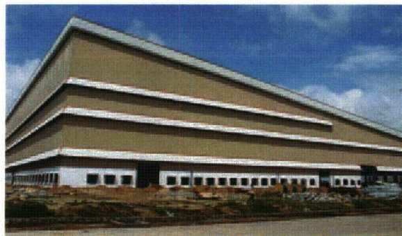
Toshiba Transmission & Distribution Systems (India) Pvt. Ltd.'s switch gear factory
