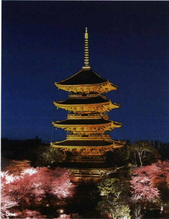
The "golden five-story pagoda" of Toji Temple in Kyoto, lit up with LED lighting
