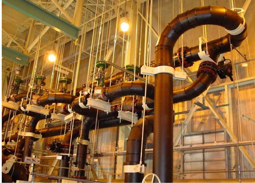
**Figure 2 Polyethylene Pipe (black piping) used at Duke Energy Catawba Plant in *non-safety* Applications**
