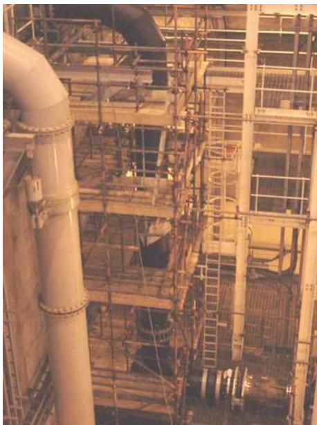
**Figure 16 – HDPE pipe (black) installed at Sizewell B by British Energy**
