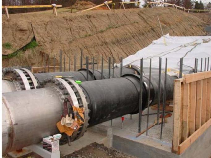
**Figure 15 Flanged connection from HDPE to steel piping
