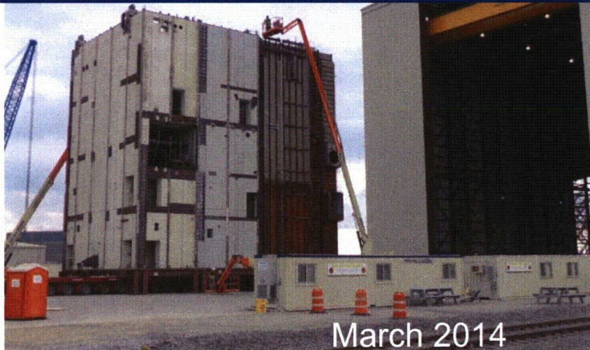
Aux. Bldg. Structural Module (CA20 – Vogtle Unit 3)
