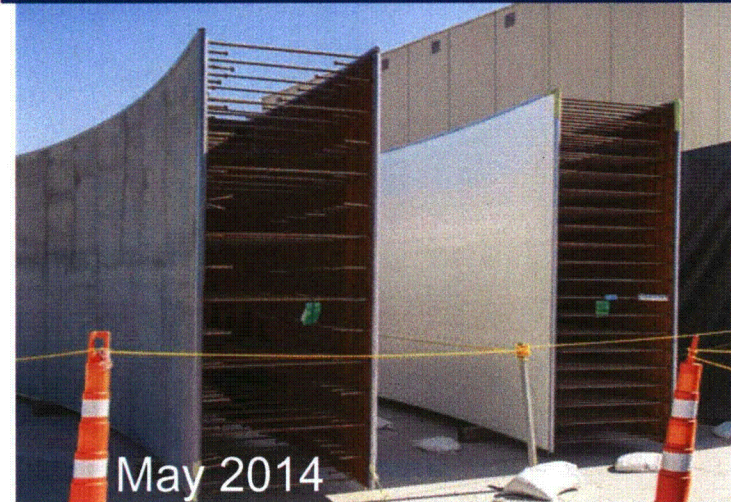
Shield Building Panels (Vogtle Unit 3)
