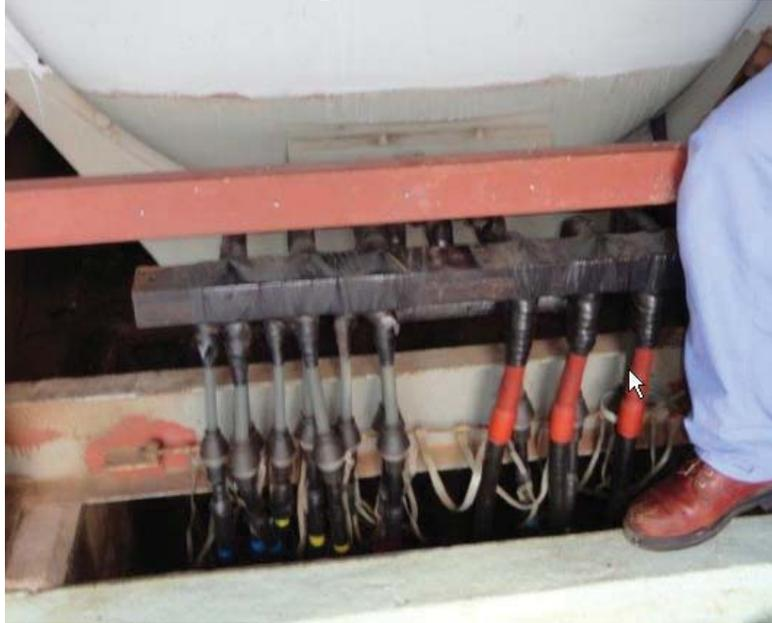
Emergency Diesel Generator output cables (Plant safety related DG's). Conceptual, other connection options are being evaluated.
