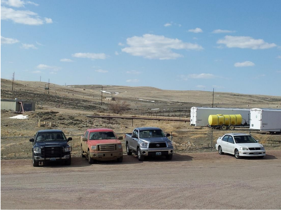
Looking South Over Cameco Wellfield
