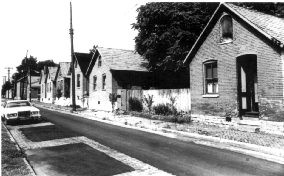
The German Village Historic District in Columbus, Ohio, reflects the ethnic heritage of 19th century German immigrants. The neighborhood includes many simple vernacular brick cottages with gable roofs. (Christopher Cline)
