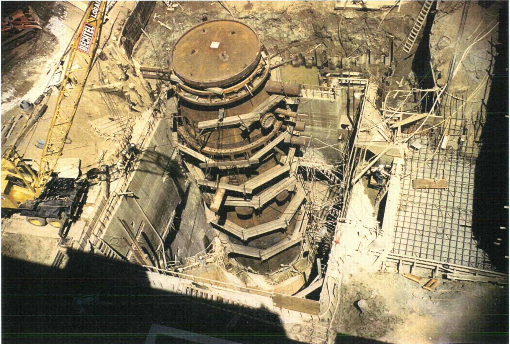
Reactor Drywell in Place
