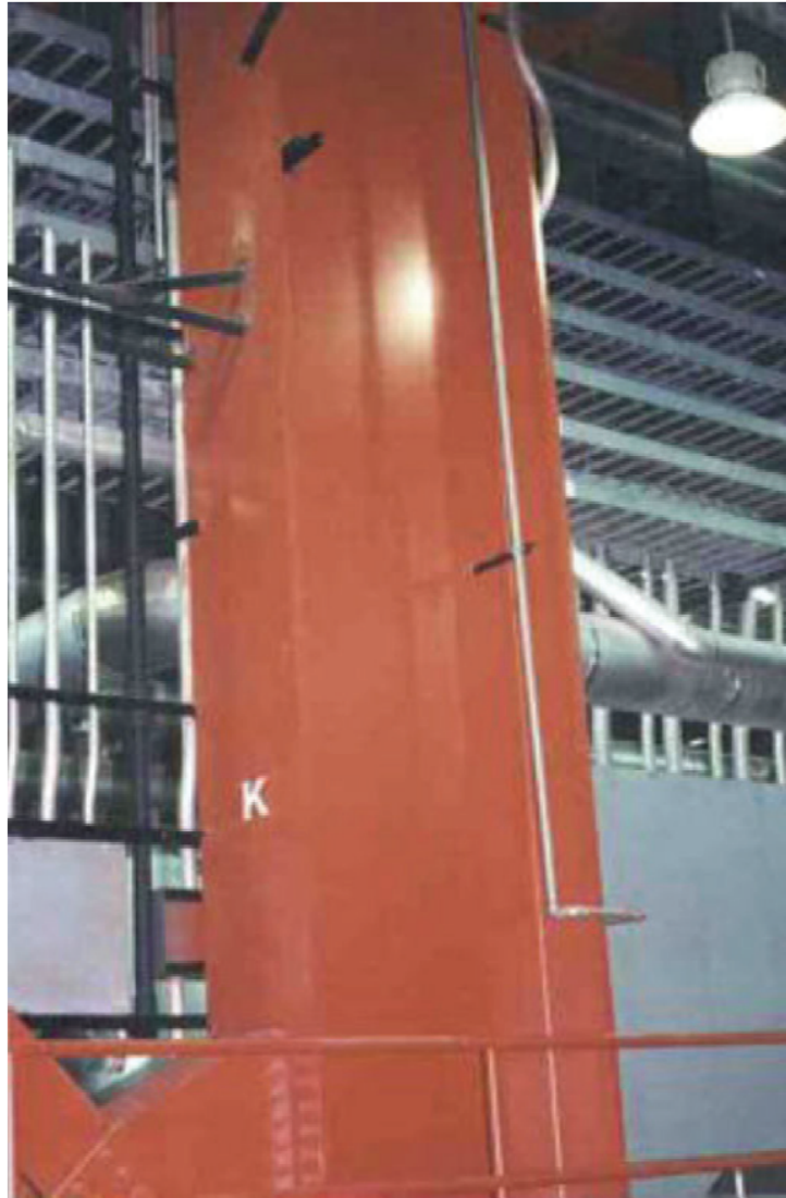
Figure F-2. Structural Steel Column in the Turbine Building.
