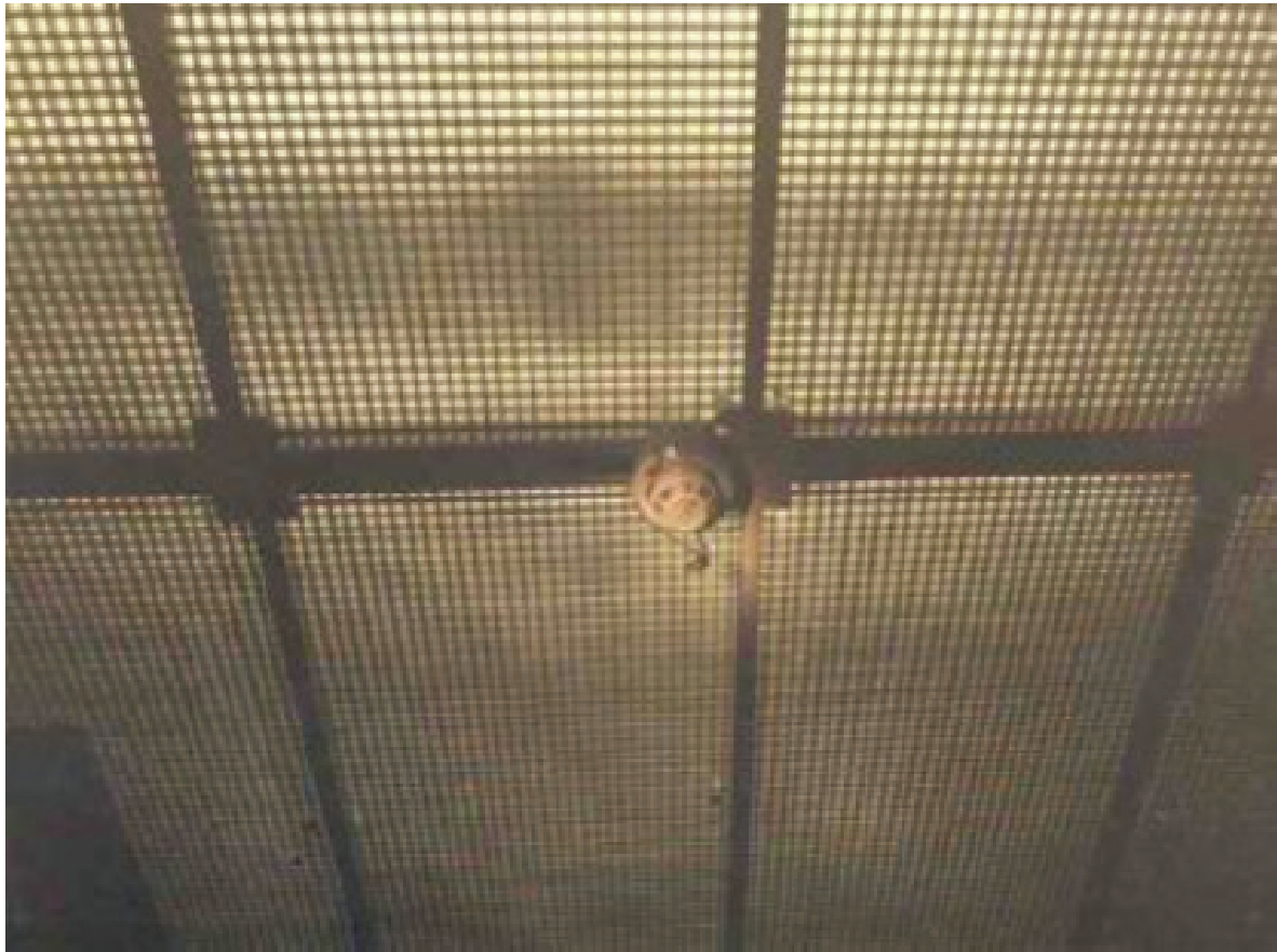
Typical “open grate” ceiling
