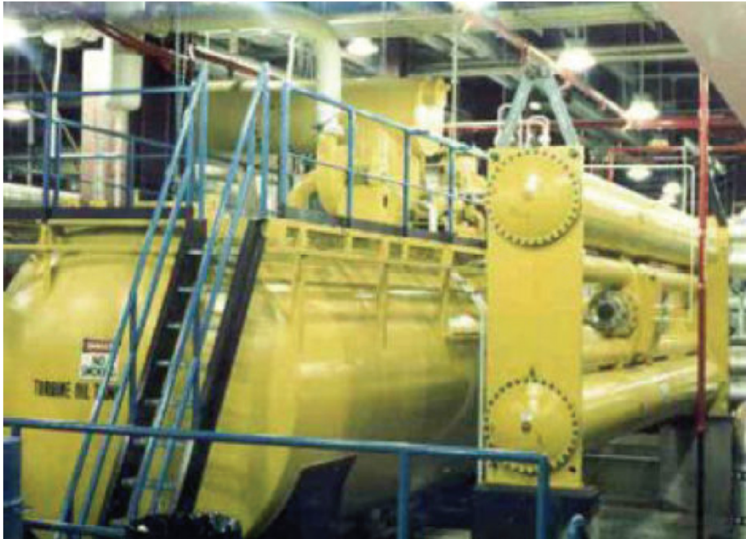
Figure F-3. Main Turbine Lubricating Oil Tanks in the Turbine Building.
