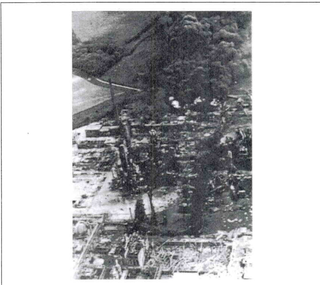
Fig. 6. VCE at Flixborough Plant
