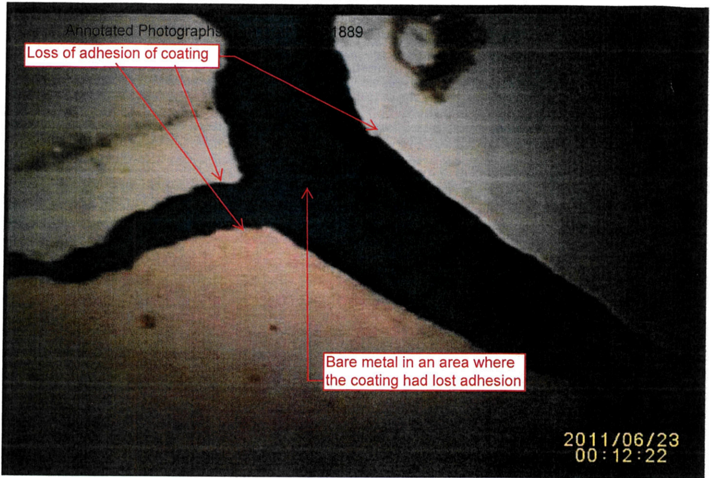
From CAP 01291889, Bottom Inspection of Cask #1
