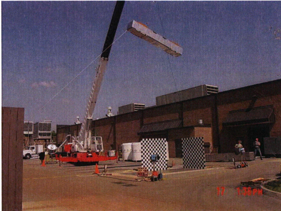
Figure 2-25 CTU 1 Positioned for 15° 9-m (30-foot) Slap-down Drop
