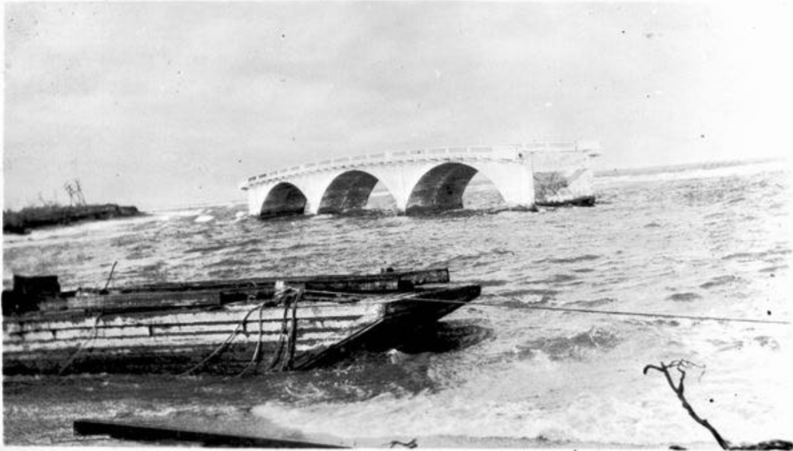
Figure 20. Remains of the bridge at Bakers Haulover Cut after the Hurricane of 1926. (See Figure 12 for aerial photograph of bridge before the hurricane.) [Photo negative, black and white 4 x 5 in. N031942. General collection, Florida State Photo Archive. < http://fpc.dos.state.fl.us/ >]
