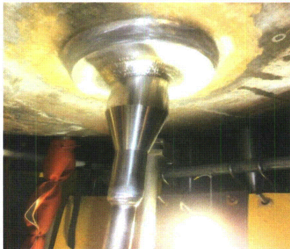
Figure 4 - Drawing of Repaired Unit 3 BMI Nozzle 3
