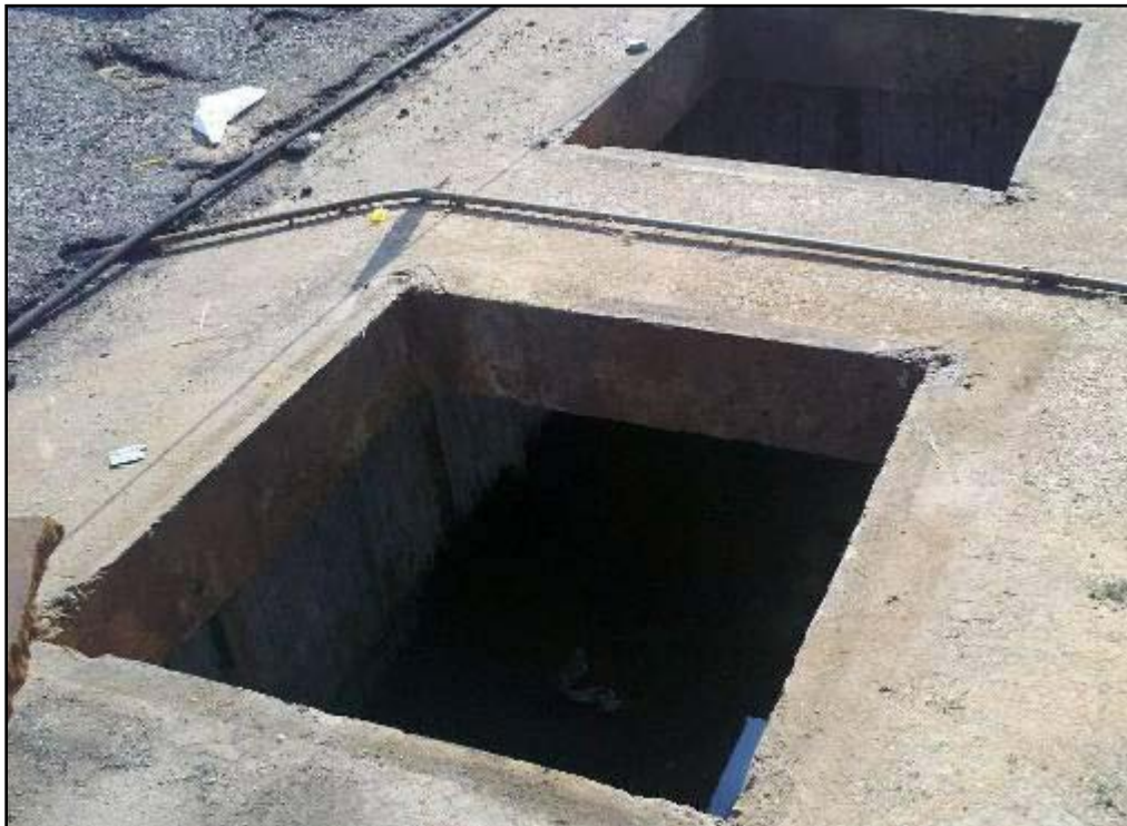
Figure 33-3 Photograph of Access to the Weir Chamber Looking West
