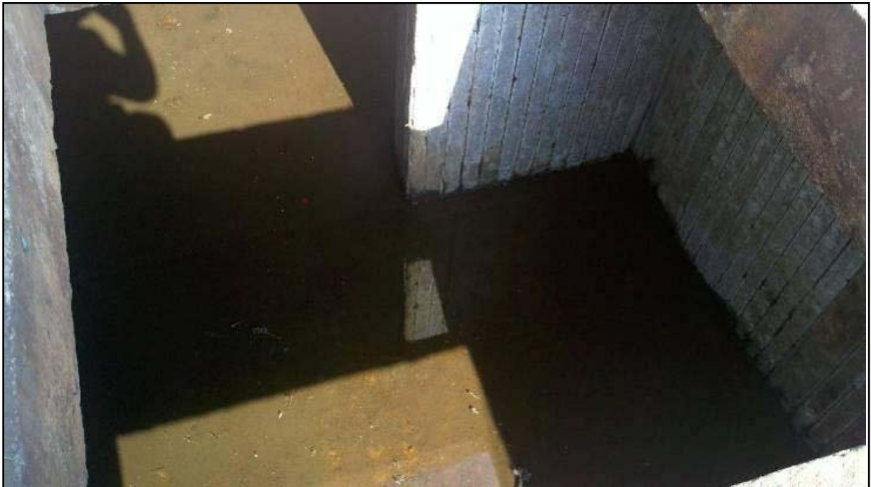
Figure 33-5 Photograph of Main Section of Weir Chamber Looking East
