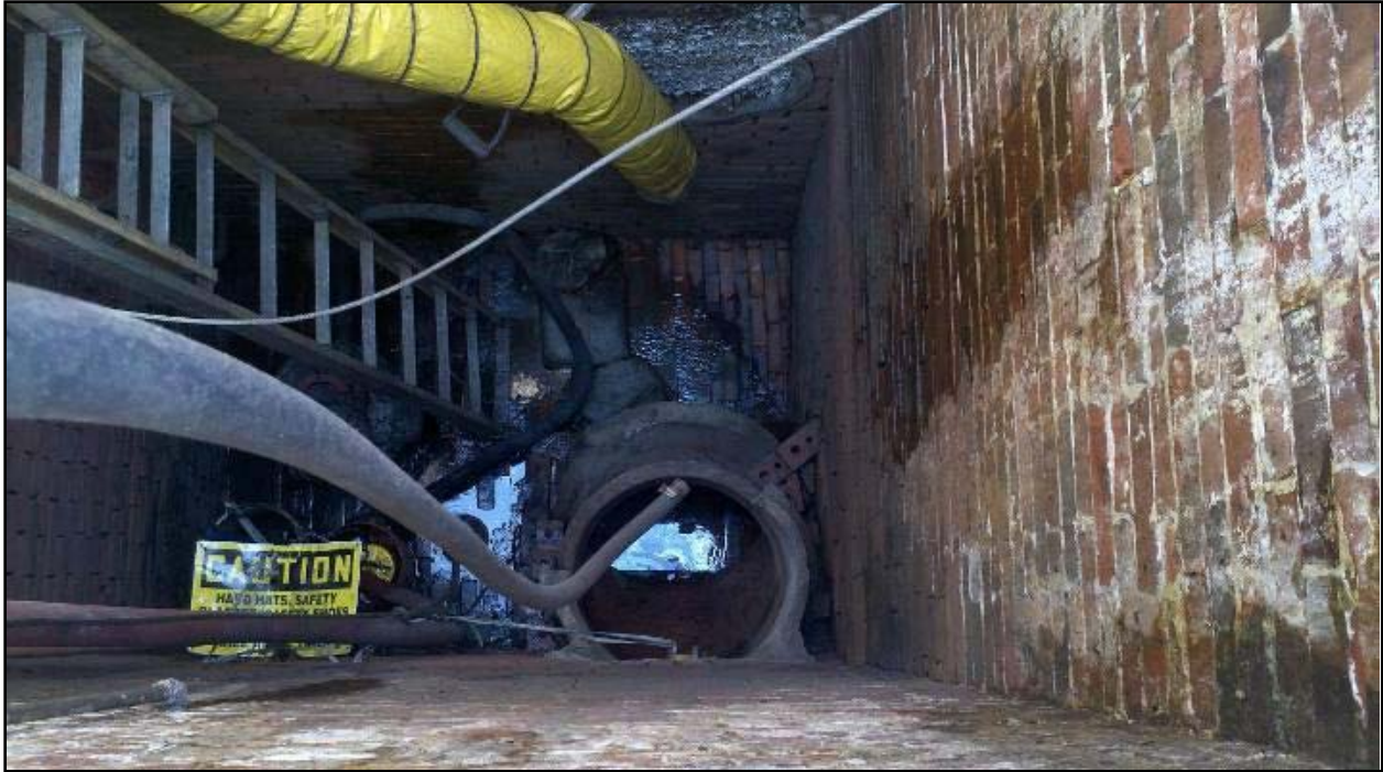
Figure 33-11 Photograph of Pump Vault Looking East
