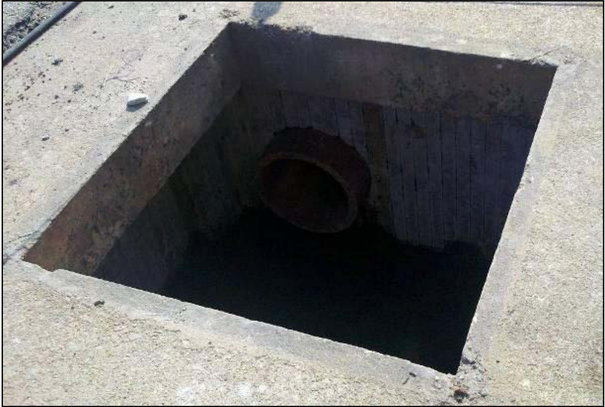
Figure 33-4 Photograph of 12-inch Pipe at Bottom of the Weir Chamber
