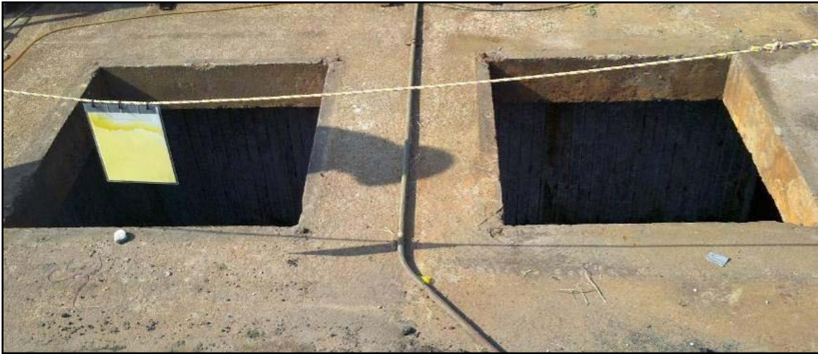
Figure 33-2 Photograph of Access to the Weir Chamber Looking North
