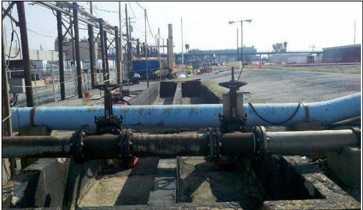
Figure 33-8 Photograph of Grit Chamber Looking East
