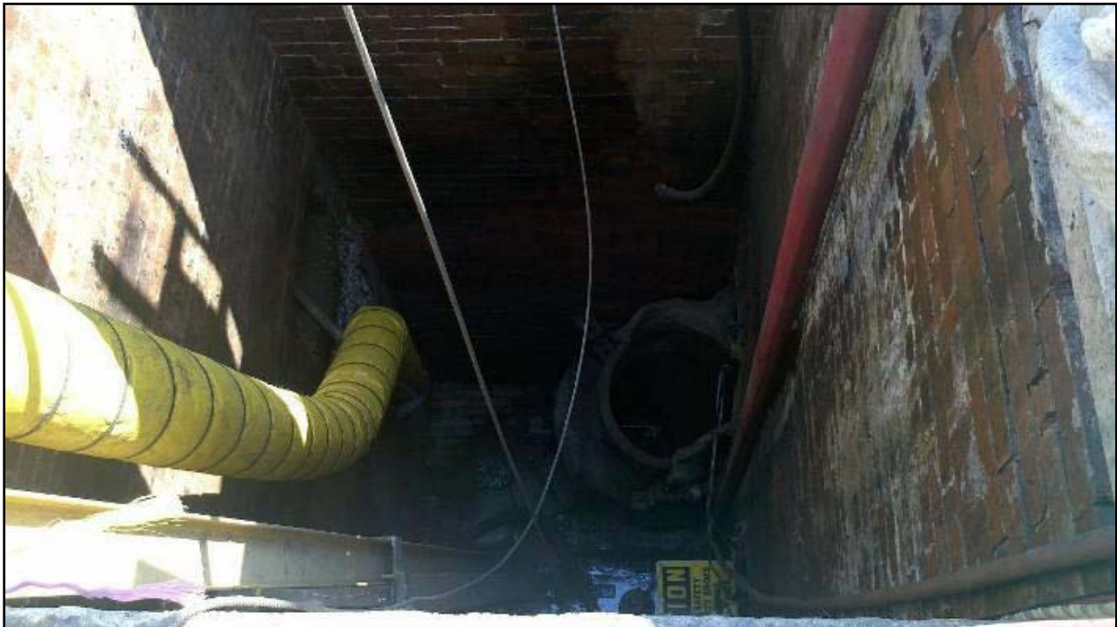
Figure 33-12 Photograph of Pump Vault Looking South
