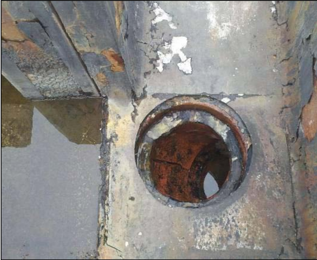
Figure 33-10 Photograph of Southeast Drain of Grit Chamber
