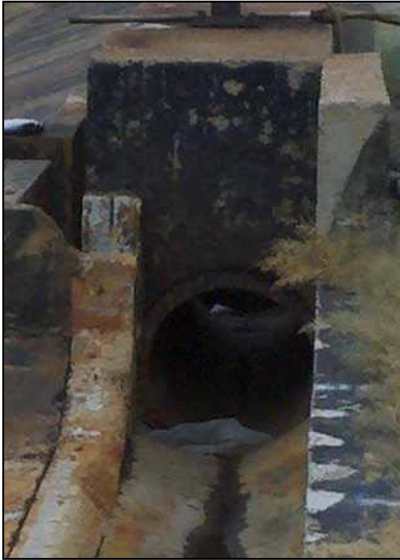
Figure 32-7 Photograph of Northern Trough Connection Pipe
