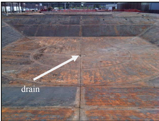
Figure 32-5 Photograph of Plant 7W West Basin Looking East
