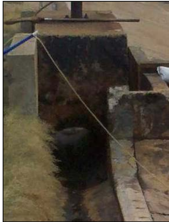
Figure 32-8 Photograph of Northern Trough Connection Pipe
