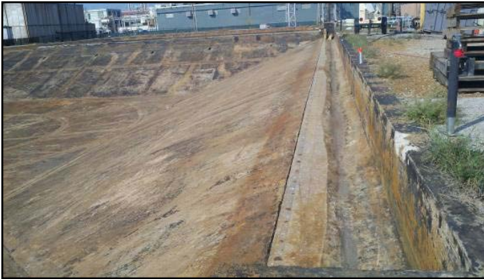
Figure 32-4 Photograph of Plant 7W East Basin Northeast Corner Looking West
