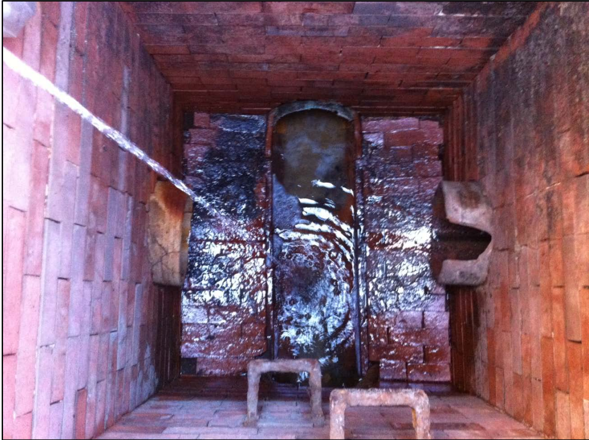
Figure 29-2 Photo of Manhole MH-X
