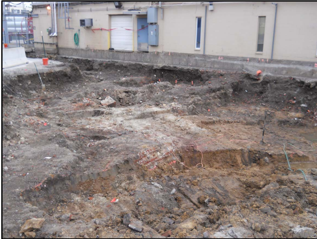
Figure 28-7 Photograph (3) of SU10 West Wall – South End (Building 240)
