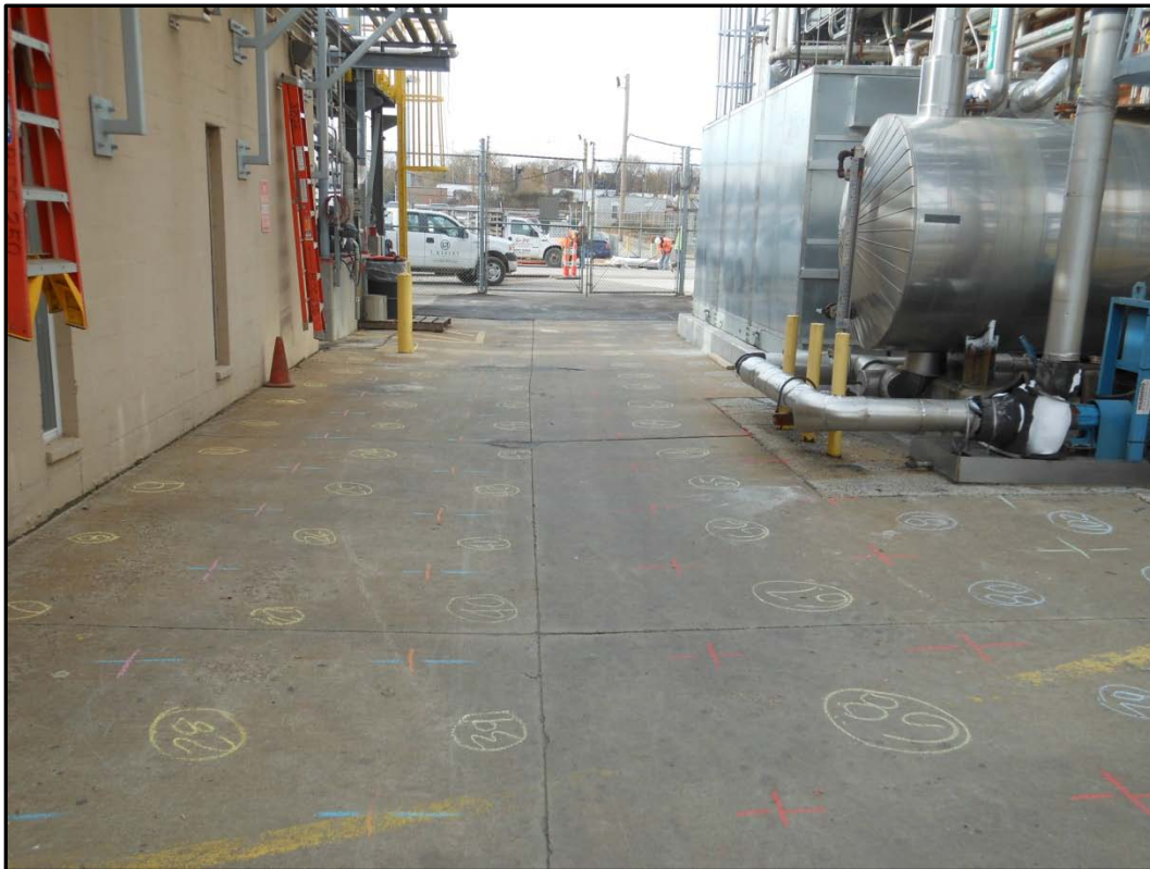
Figure 28-3 Photograph (1) of SU22 – Building 240/250 Alley (West View)
