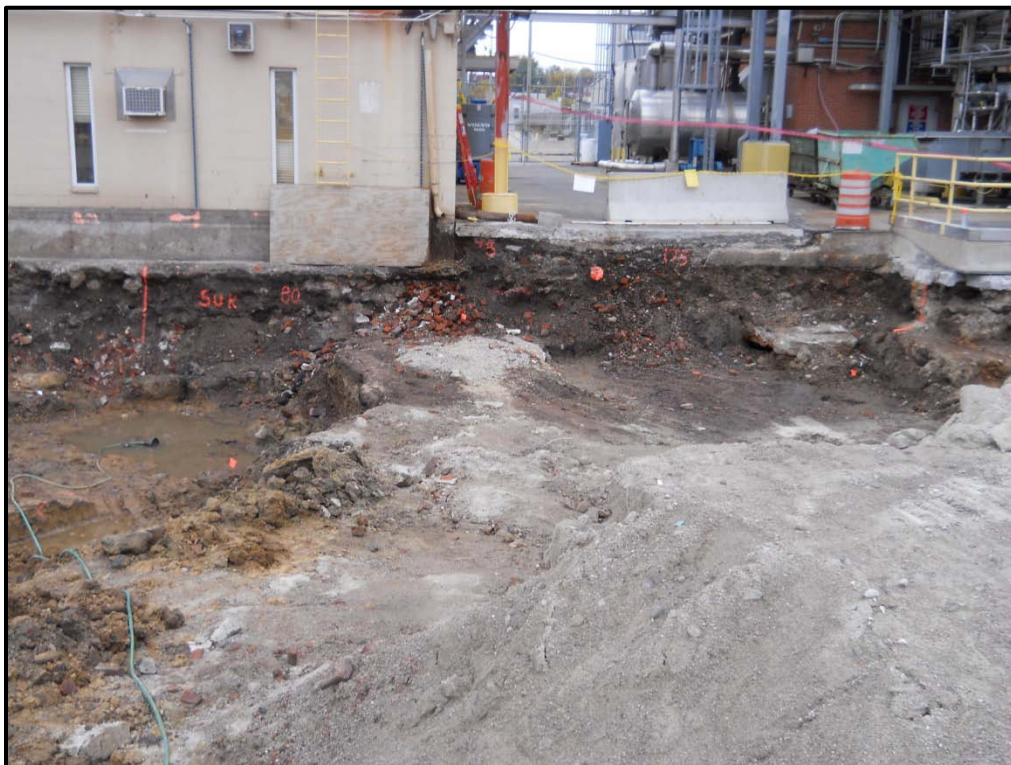
Figure 28-8 Photograph (4) of SU10 West Wall – North End (Building 240/250 Alley)
