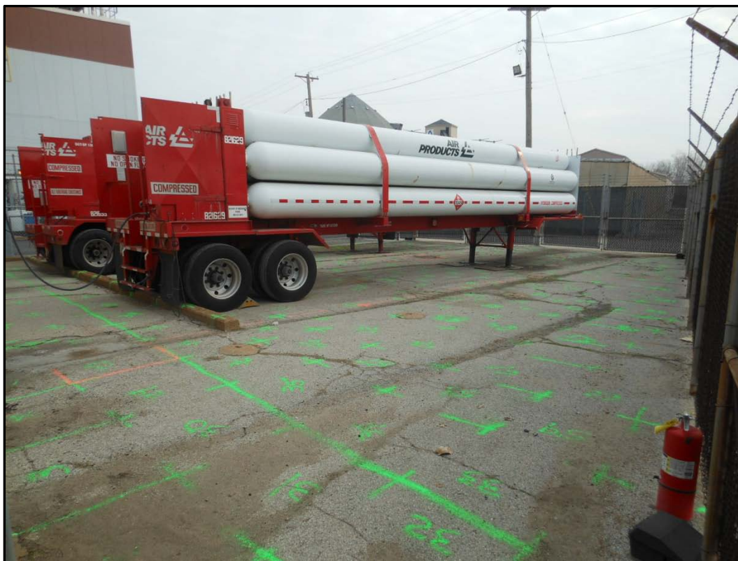
Figure 28-5 Photograph (2) of SU22 – Building 240 Hydrogen Yard (SSE View)
