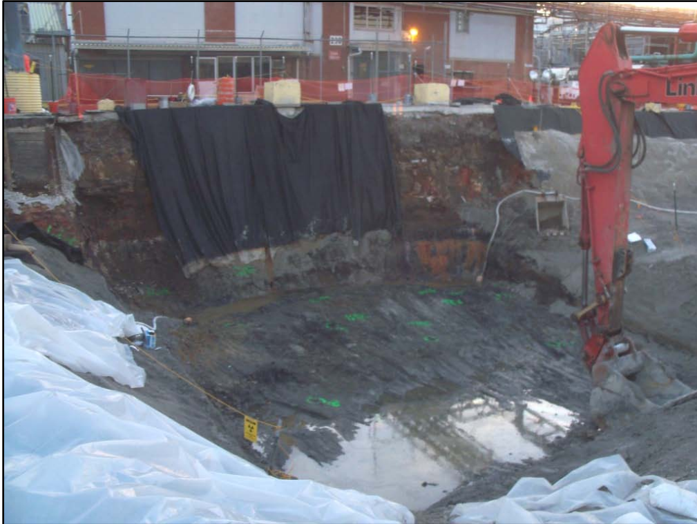
Figure 26-6 Photograph (4) of SU20 AECOM Grids E5/F5 (East View)
