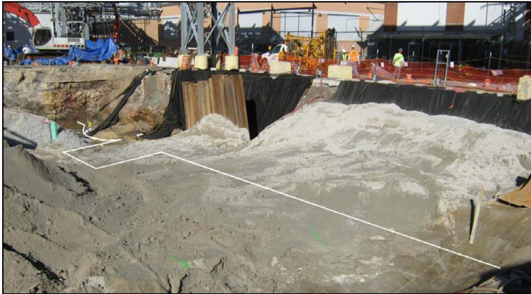
Figure 26-3 Photograph (1) of SU20 Looking East during backfill (Northeast View)
