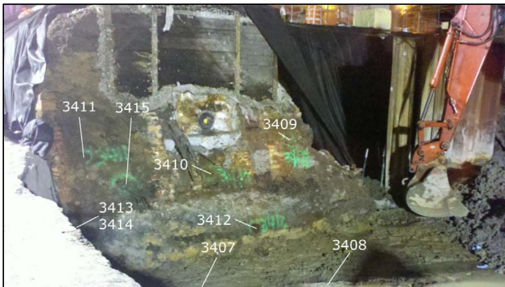
Figure 26-5 Photograph (3) of SU20 West Side of Pile Cap (East View)
