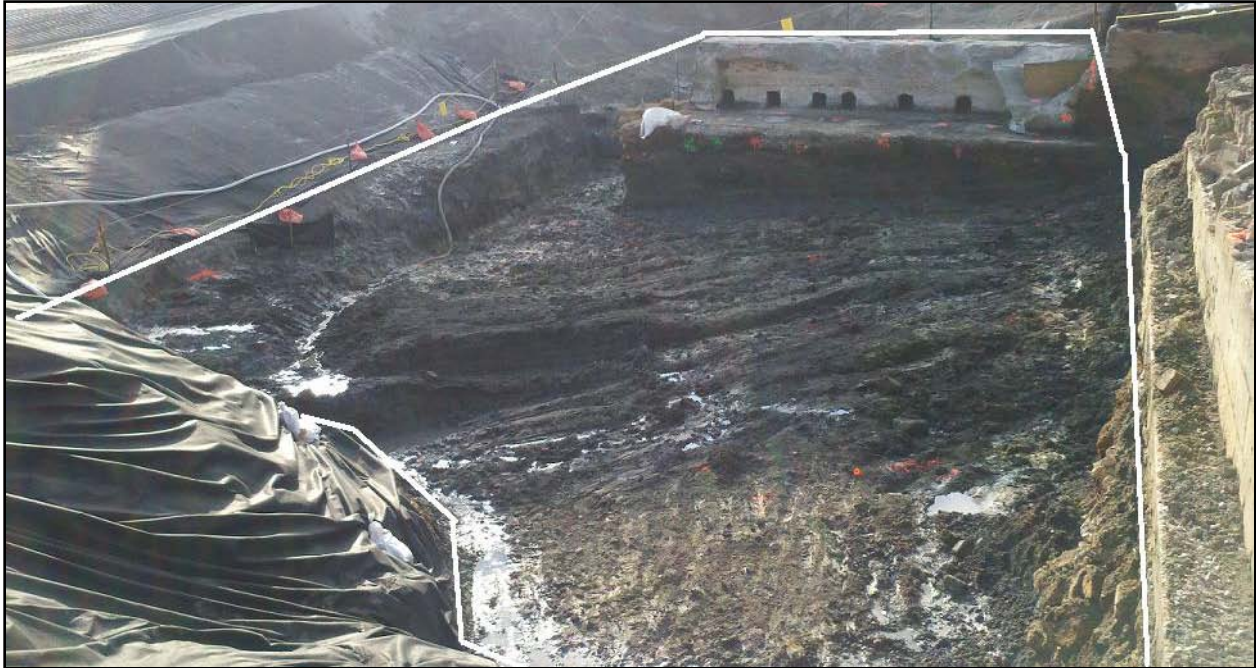
Figure 15-2 Photograph of SU09 Looking West toward East Side of Building 250
