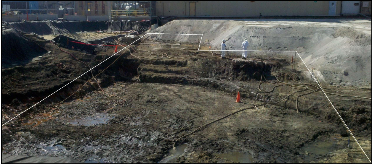
Figure 13-2 Photograph of SU07 Looking West toward East Side of Building 250
