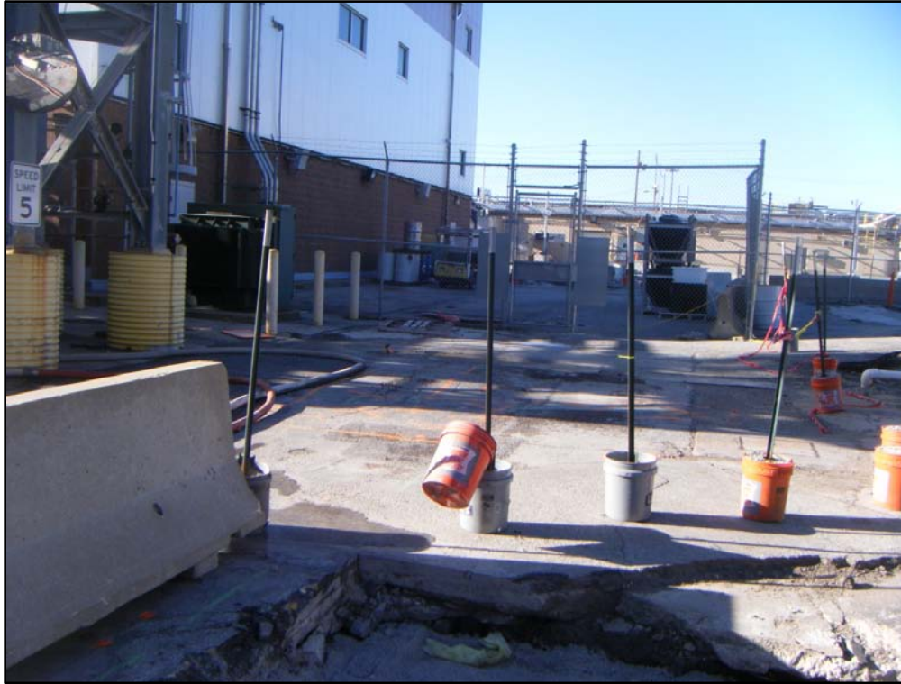
Figure 19-4 Photograph (2) SU13 North Side Building 260
