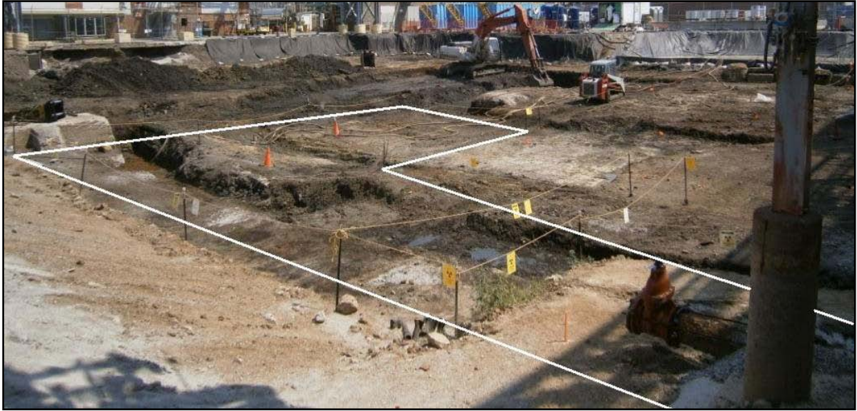
Figure 12-2 Photograph of SU06 Looking Southeast from East Side of Building 250
