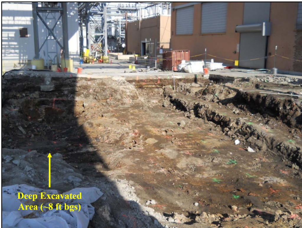
Figure 17-4 Photograph (2) of SU11 at Time of FSS (North View)
