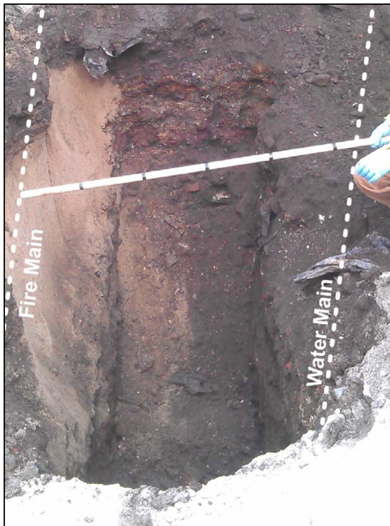
Figure 17-6 Photograph (4) of the Deep Excavation for Systematic Sample Location 7
