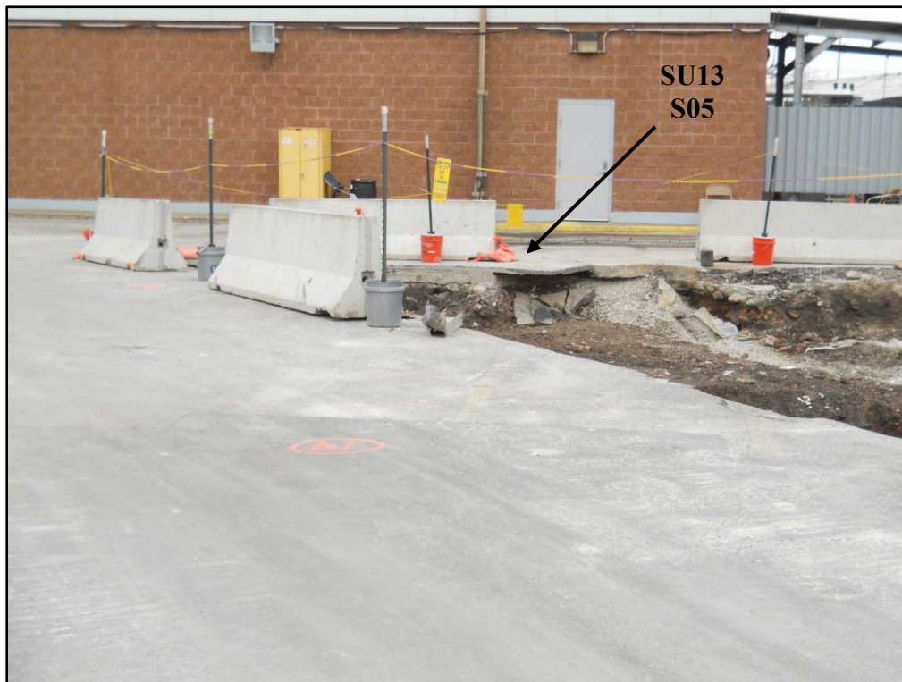
Figure 16-6 Photograph (4) of SU13 Systematic Sample Location 5
