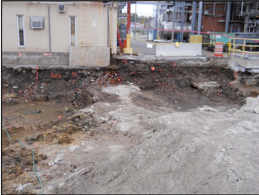
Figure 16-11 Photograph (6) of SU10 West Wall – North End
