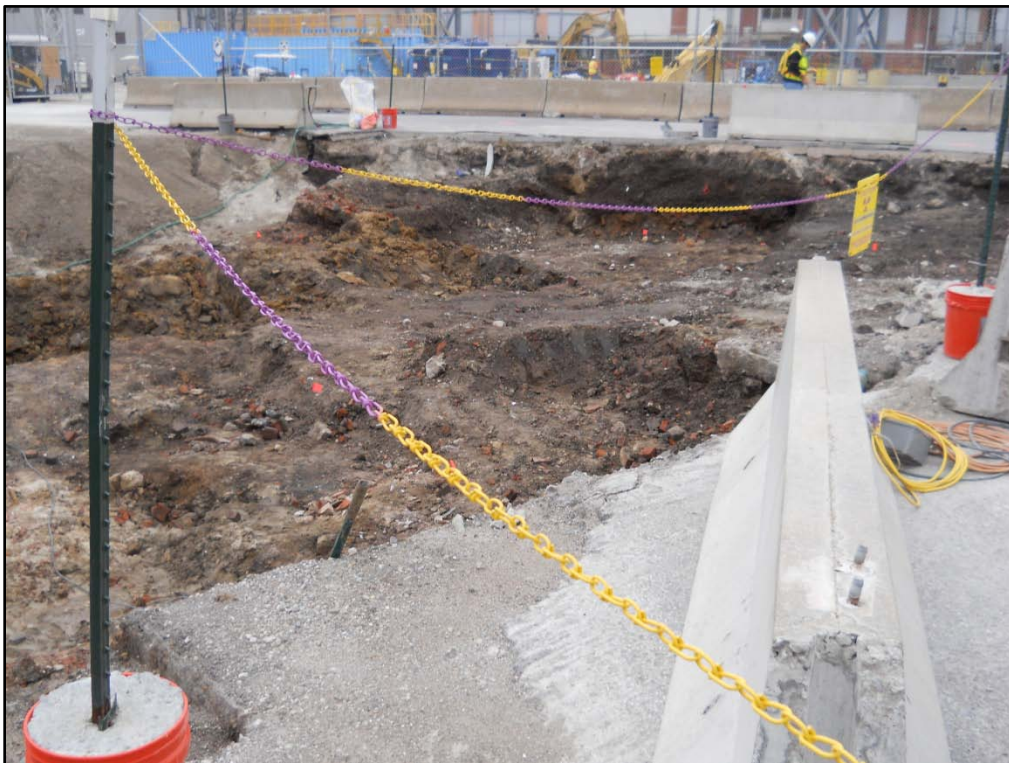
Figure 16-5 Photograph (3) of SU10 at Time of FSS (Northeast View)
