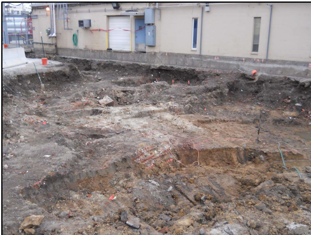
Figure 16-10 Photograph (5) of SU10 West Wall – South End
