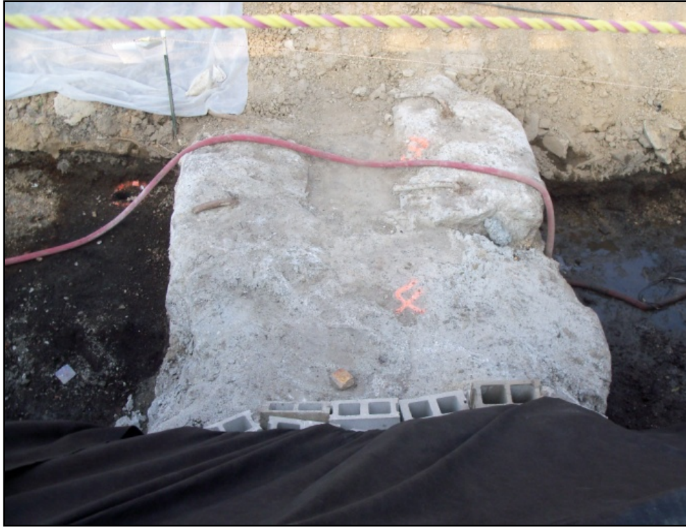
Figure 10-4 Photograph of Legacy Concrete in SU04
