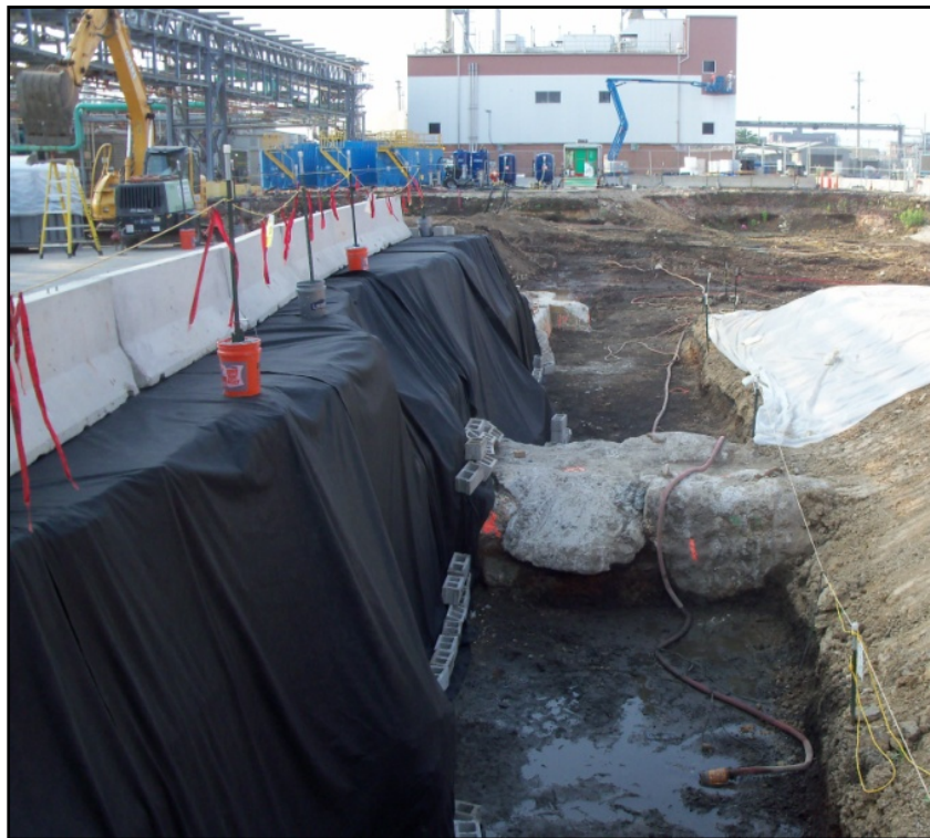
Figure 10-3 Photograph of SU04 Looking South
