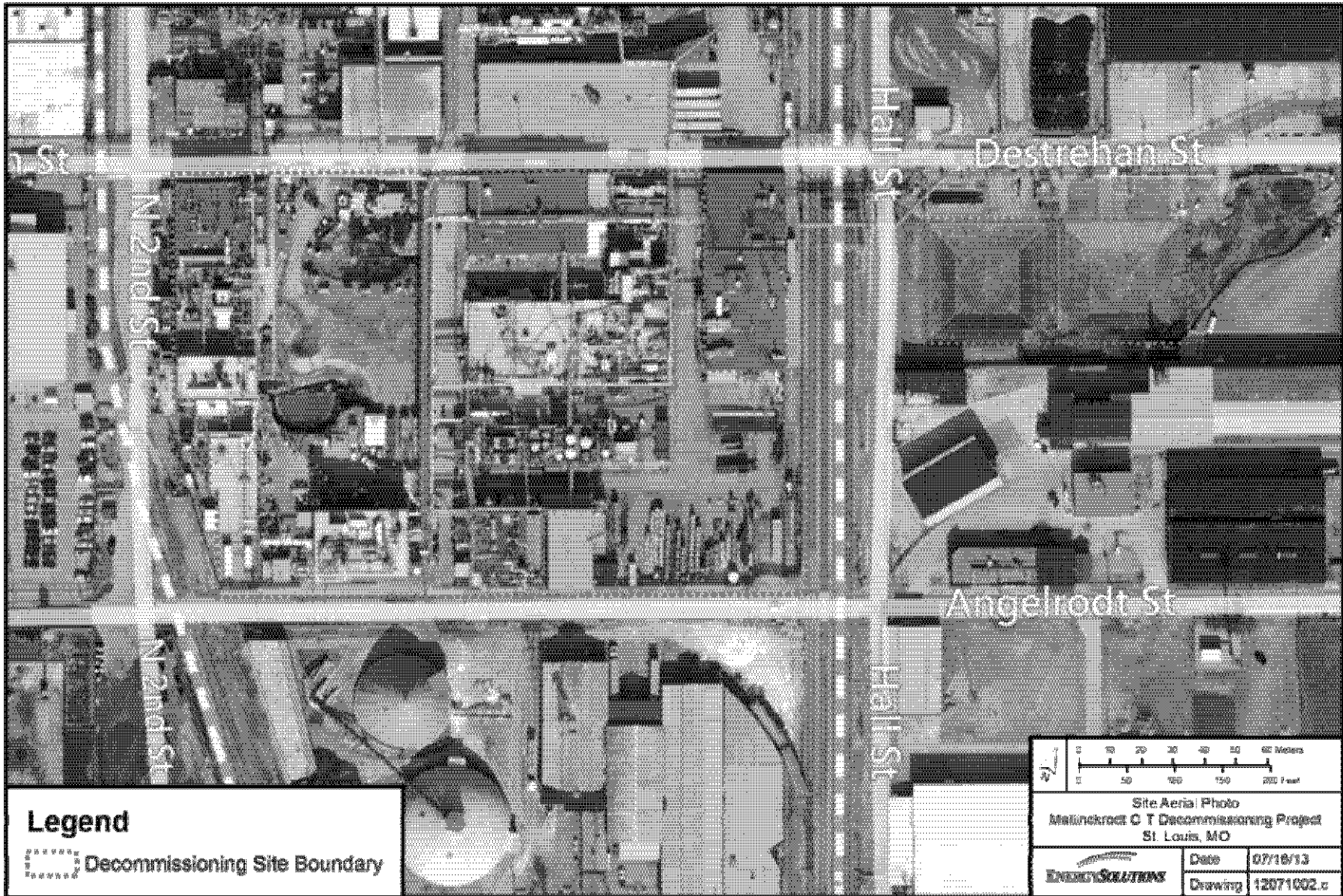
Figure 1-3 Aerial Photograph of C-T Plant
