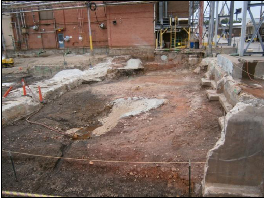
Figure 7-2 Photograph from NE Corner Looking West
