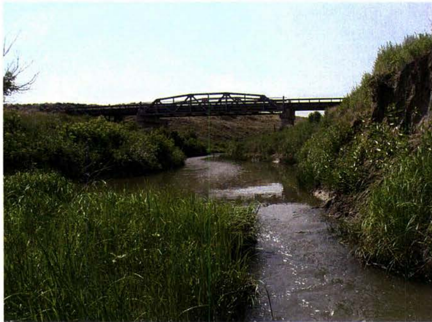
Photo 43. Site BVC04 looking upstream from Transect 8 July 8, 2008.
