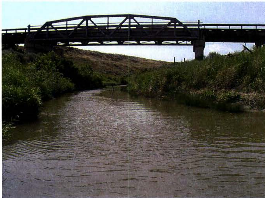
Photo 45. Site BVC04 looking upstream from Transect 10 July 8, 2008.
