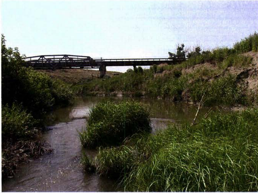
Photo 42. Site BVC04 looking upstream from Transect 7 July 8, 2008.
