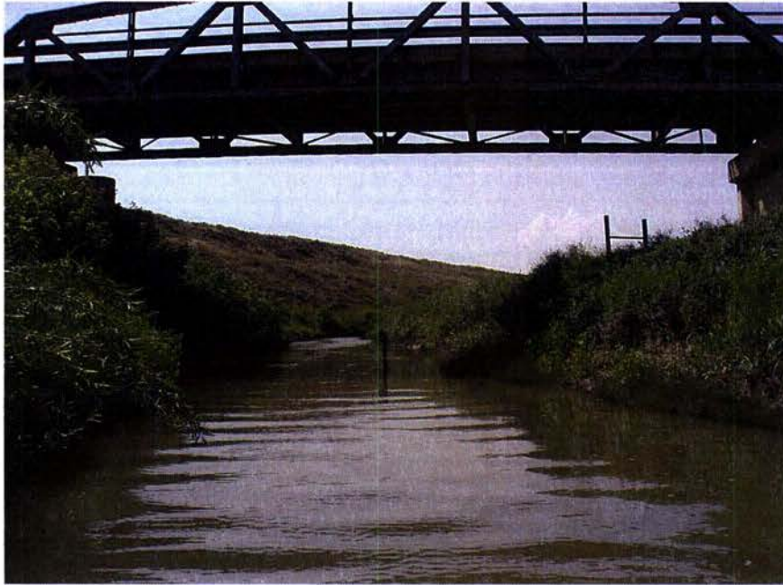
Photo 46. Site BVC04 looking upstream from Transect 11 July 8, 2008.
