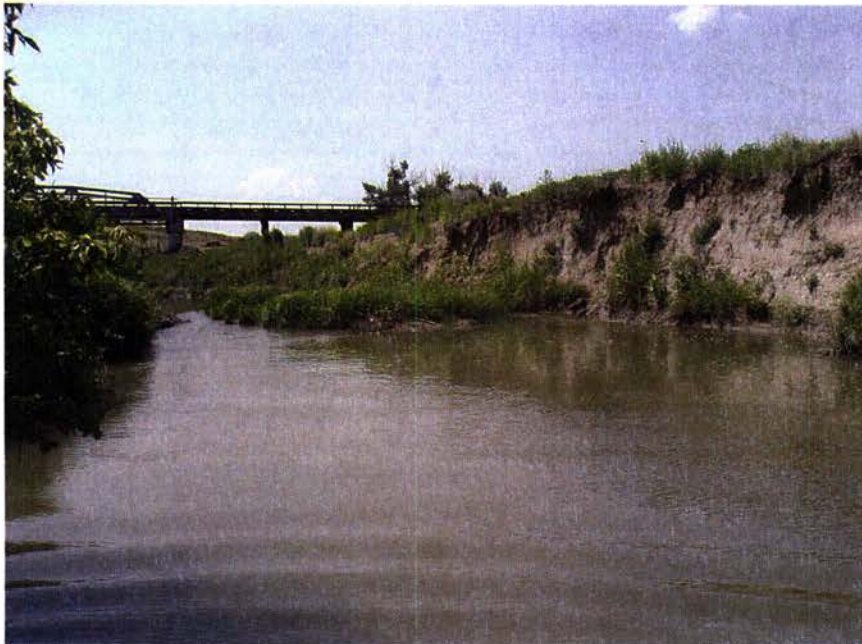
Photo 41. Site BVC04 looking upstream from Transect 6 July 8, 2008.
