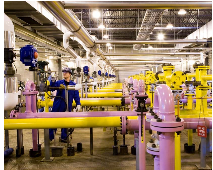
H 2 and F 2 gas lines located in UF 6 Plant at the Port Hope Conversion Facility
