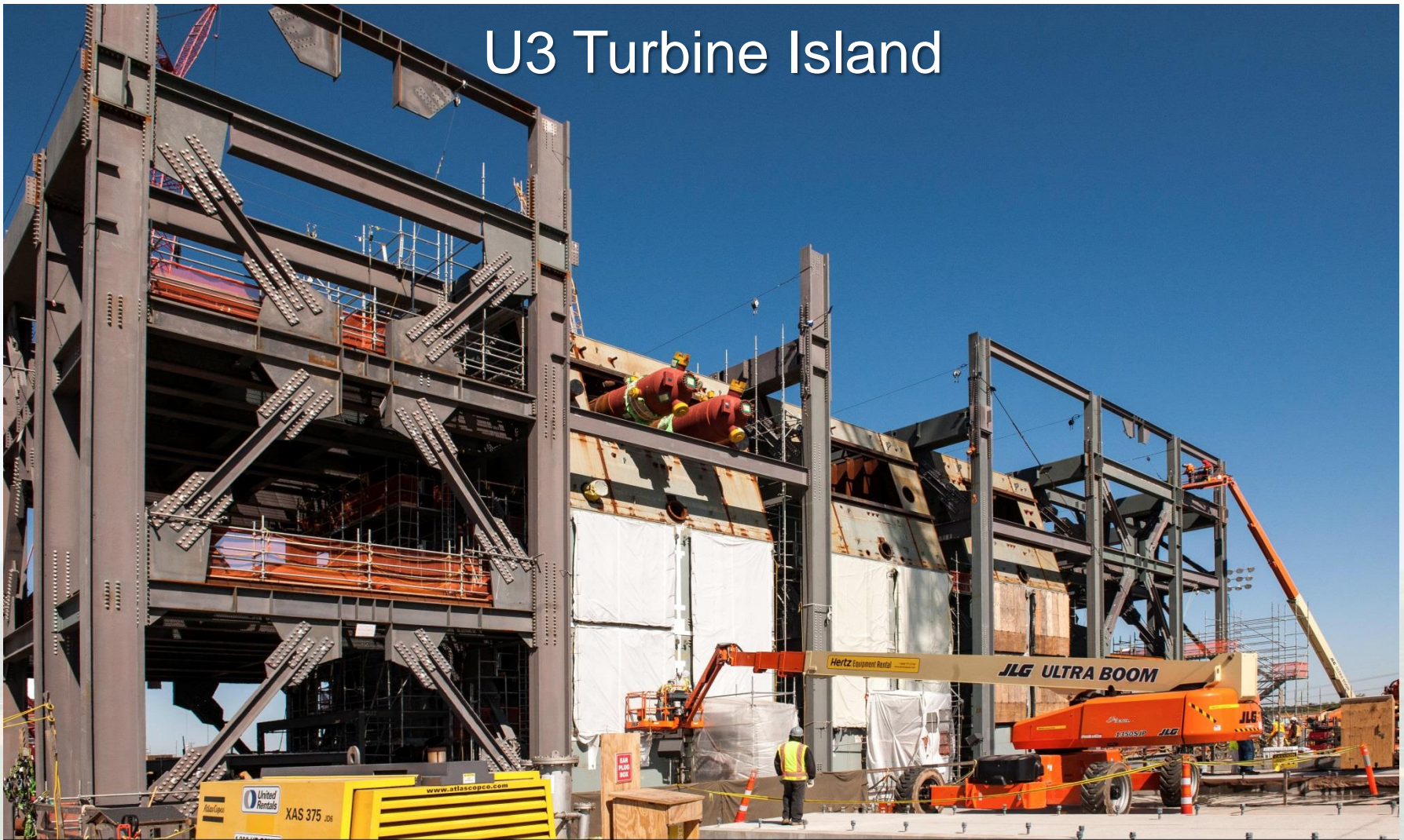
Condensers A, B and C in the Vogtle Unit 3 turbine island
