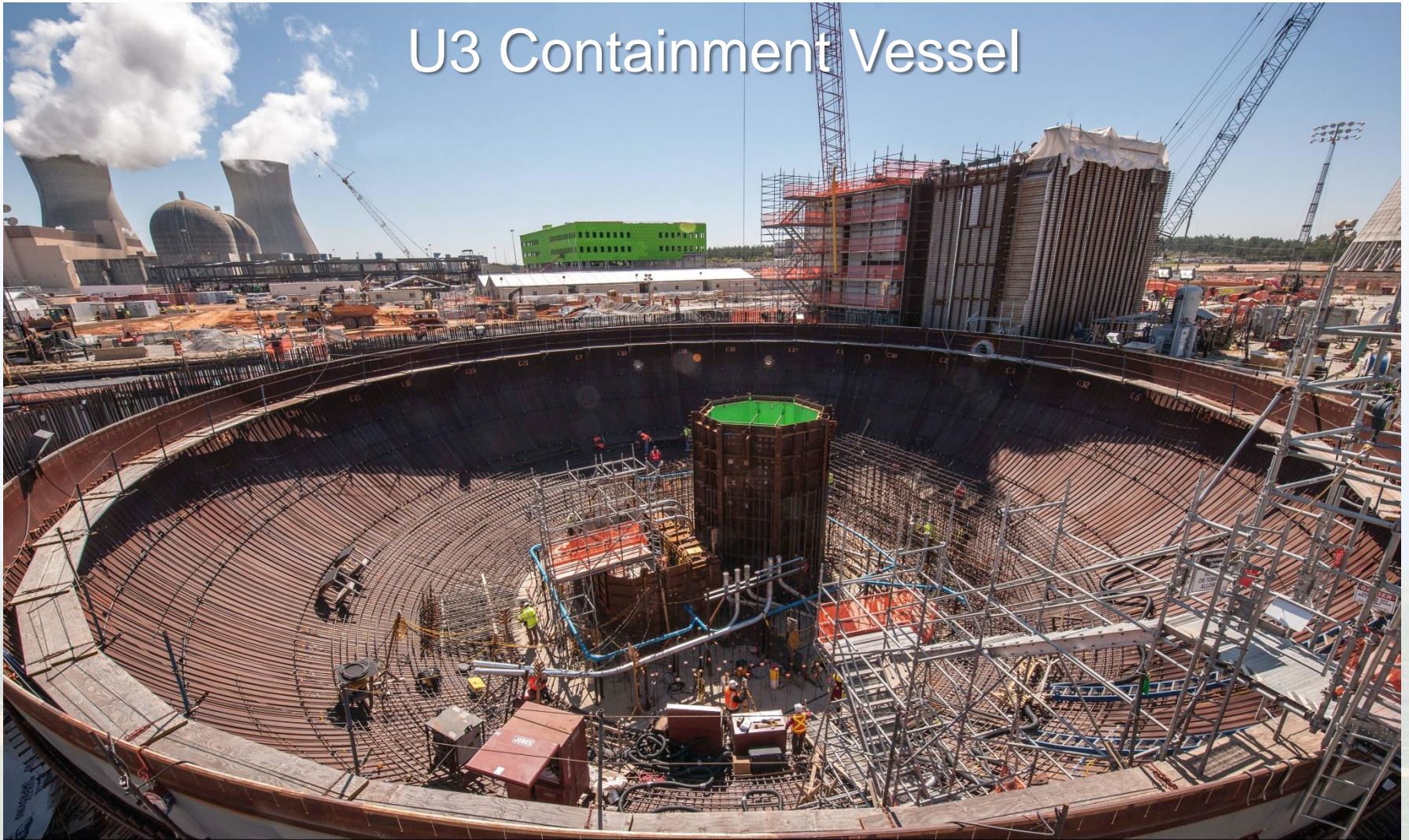
CA04 module inside the Vogtle Unit 3 containment vessel bottom head, with CA20 module in the background.
