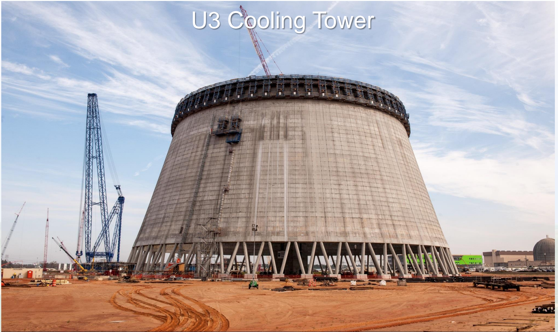
Vogtle Unit 3 cooling tower construction.
