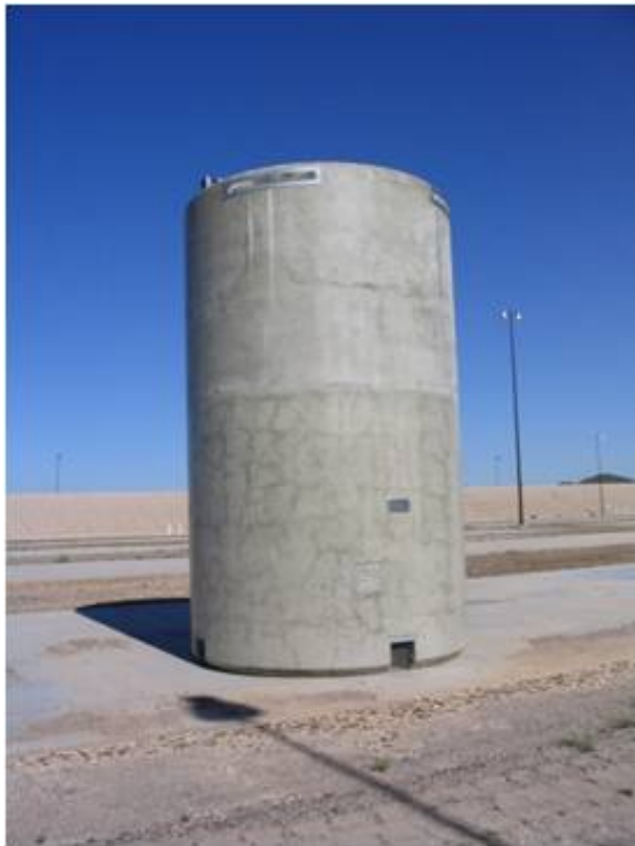
(c) Hi-Storm on Pad
