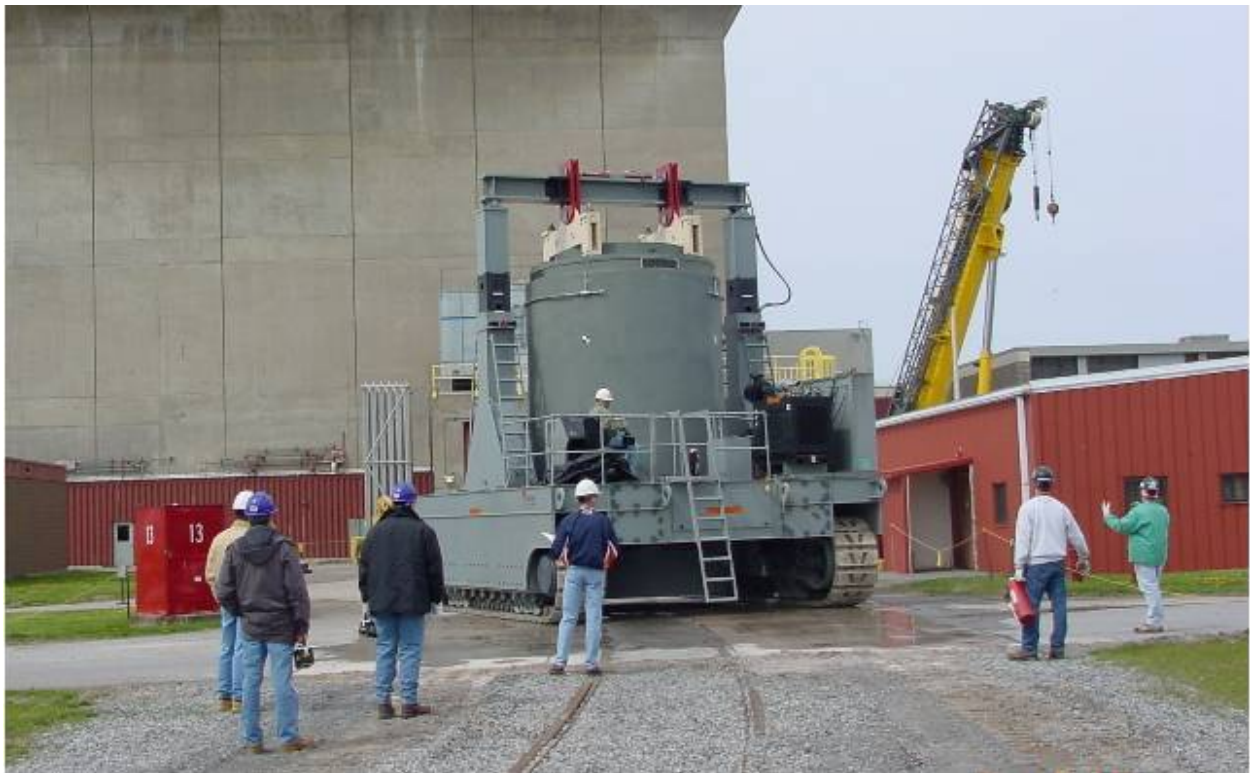
(b) Transferring Hi-Storm to ISFSI Pad
