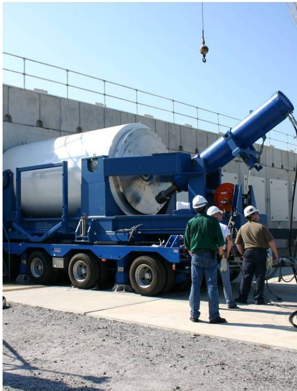
(c) Loading Horizontal Vault
