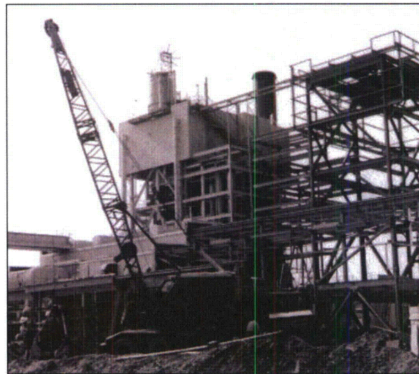
Figure 6. Construction of Unit 2 (Courtesy of PG&E)
