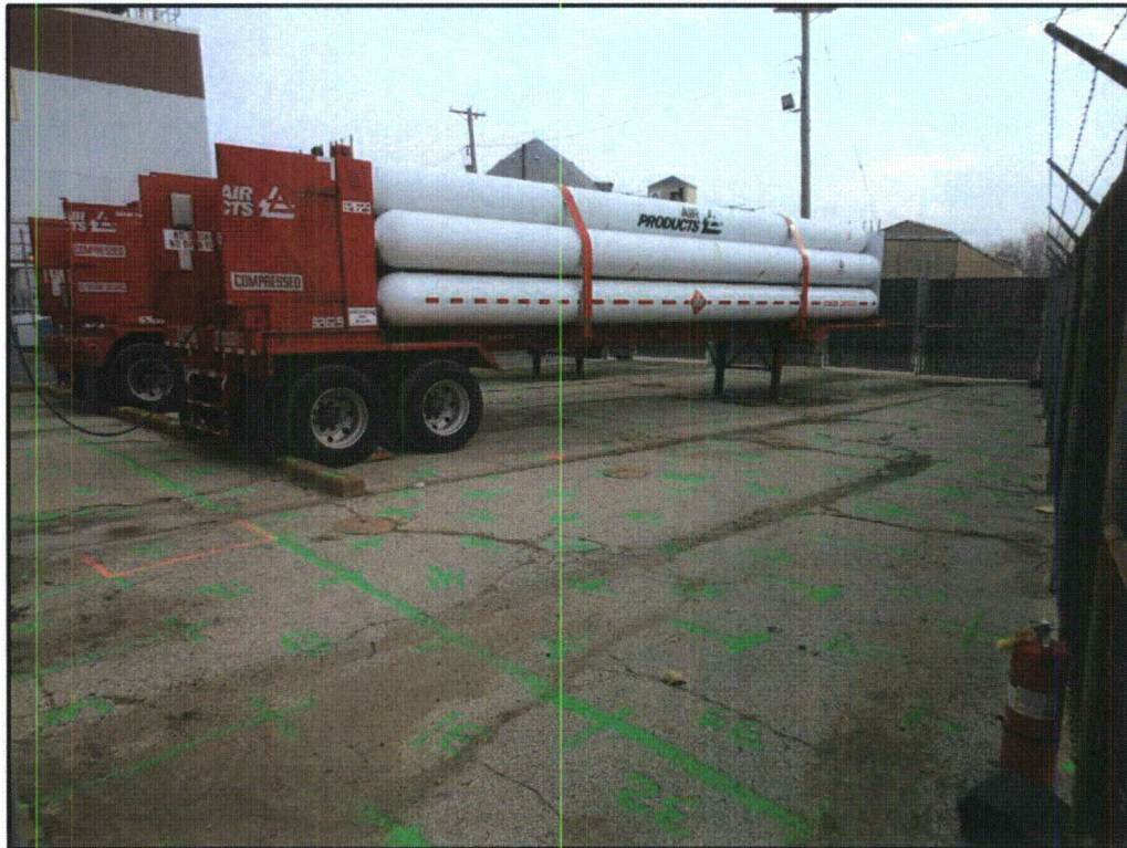
Figure 28-5 Photograph (2) of SU22 – Building 240 Hydrogen Yard (SSE View)
