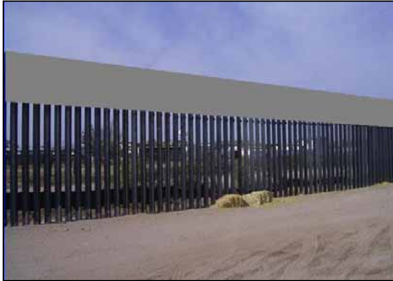
Figure 1-3. Personnel-Vehicle Fence Type 1 (PV-1)
