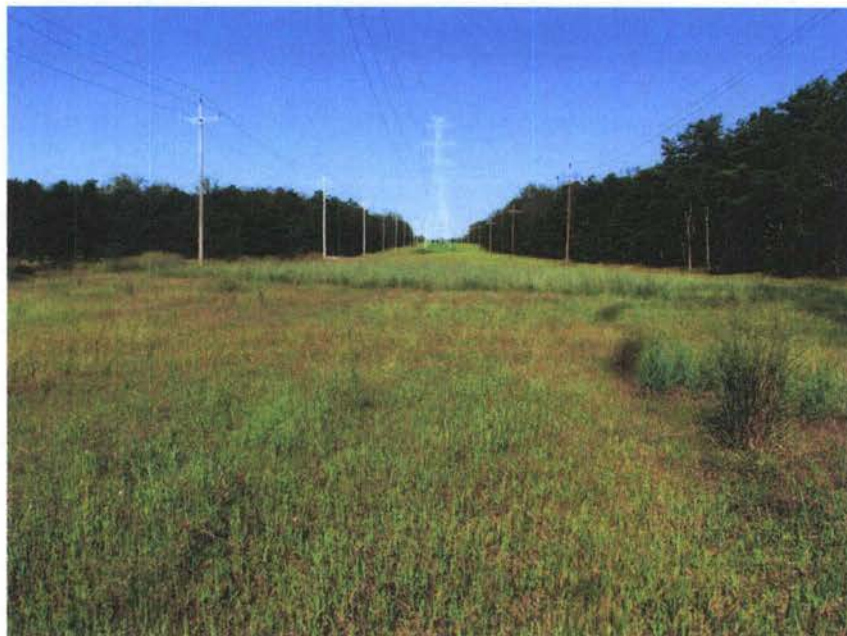
Figure 5.6. Example of span dominated by herbaceous vegetation. The span is a food plot on a New Jersey Department of Environmental Protection, Division of Fish and Wildlife, Wildlife Management Area. The vegetation-management prescription is to mow.
