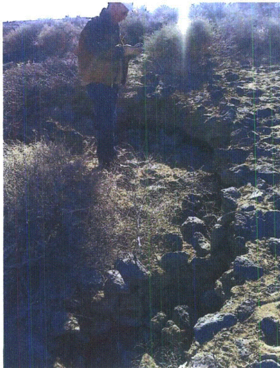
Figure 1 – LTP north slope washout viewed downslope from top of slope. Sediment in middle of picture is below the zone of concern.
