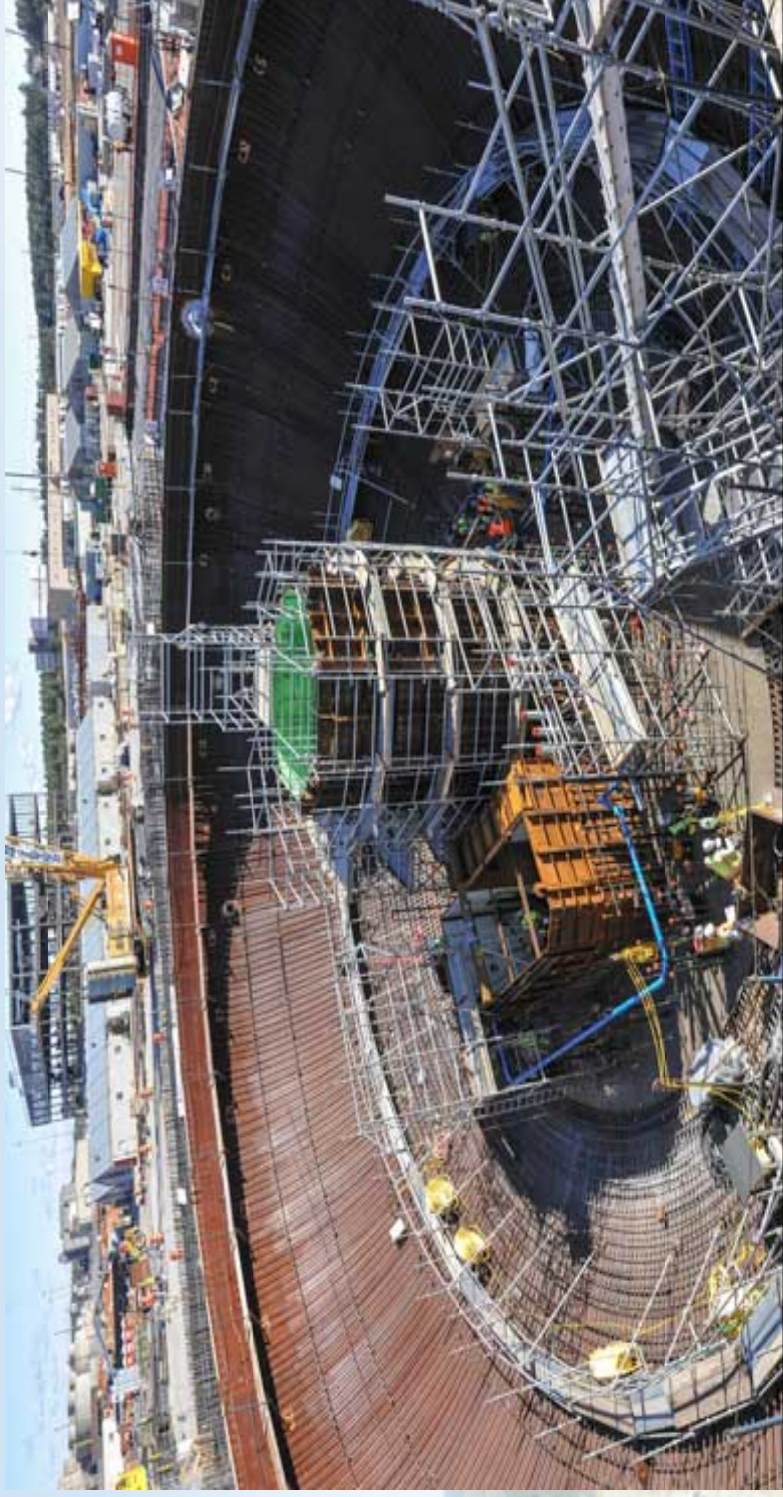
CA-04 module inside the Vogtle Unit 3 containment vessel bottom head
