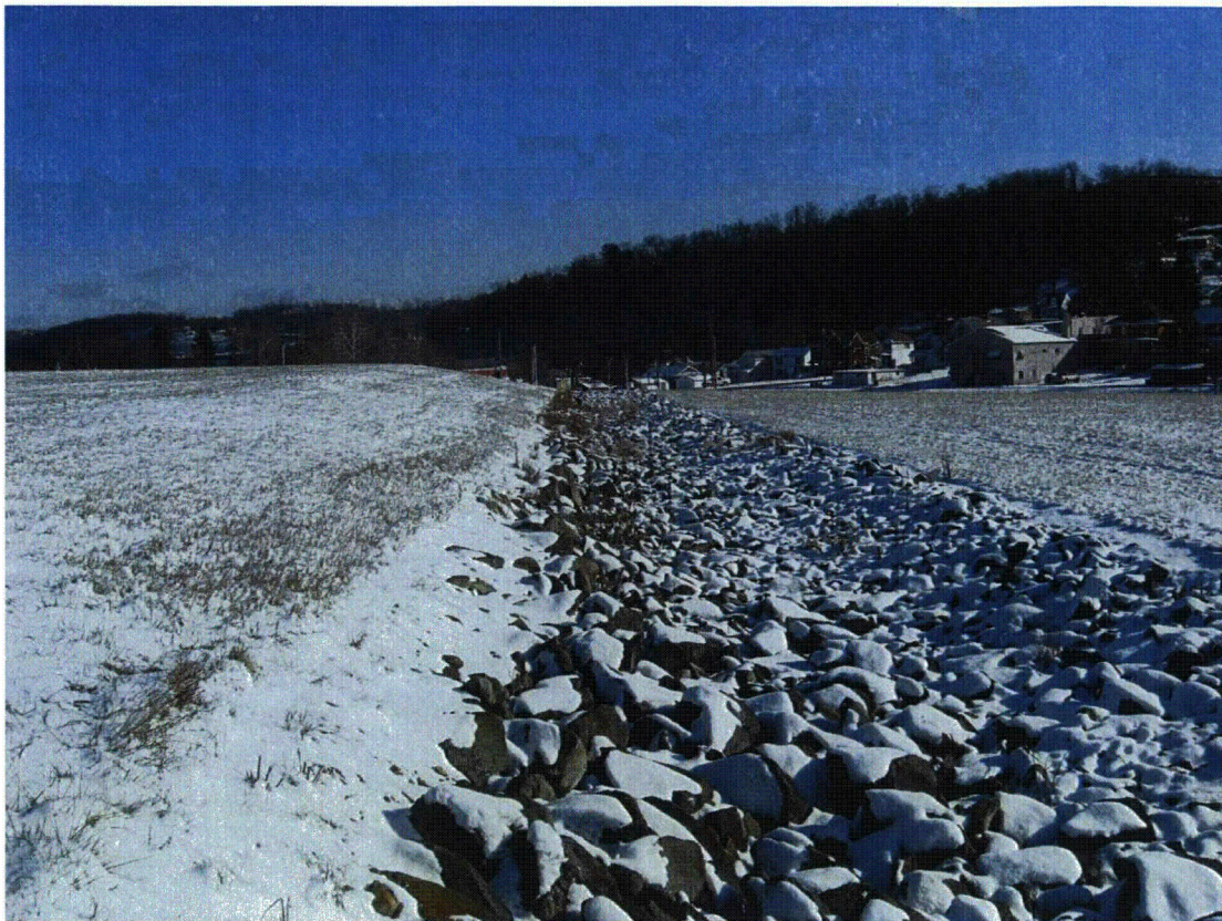
CAN 10/2013. PL-11. Riprap-armored diversion ditch on northwest side of disposal cell.
