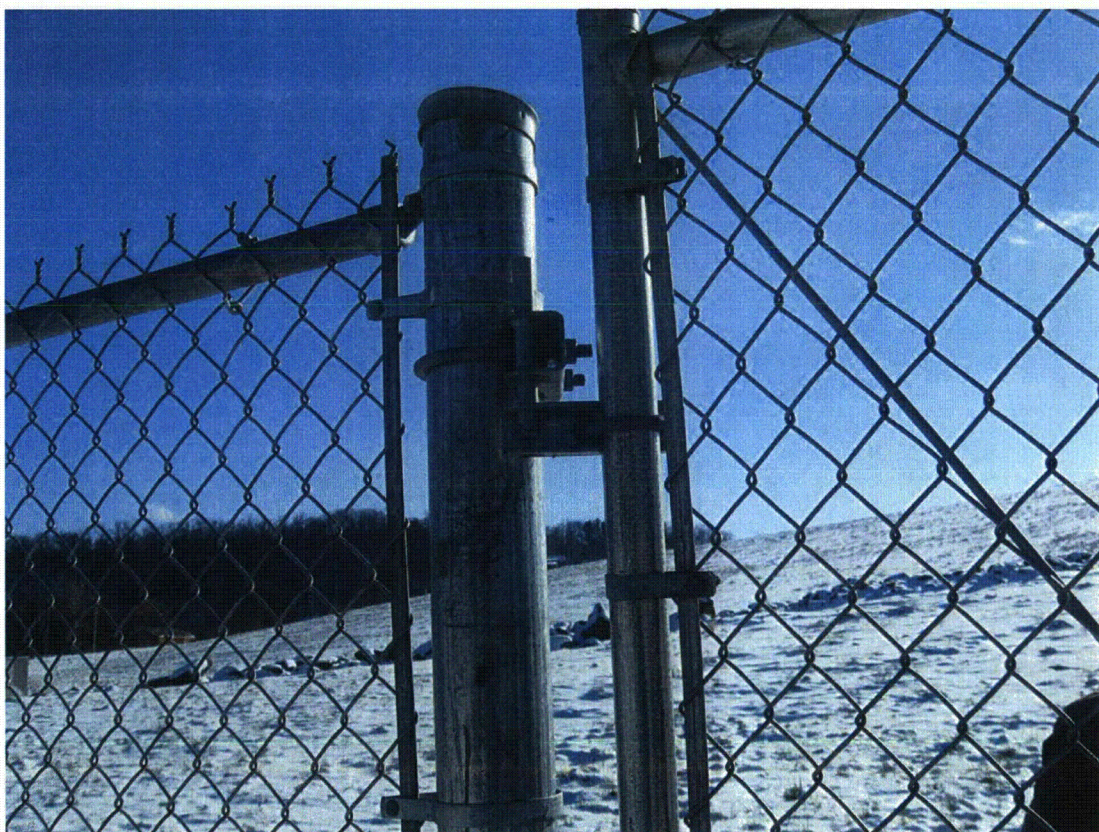
CAN 10/2013. PL-2. Damage to vehicle gate near perimeter sign P8.
