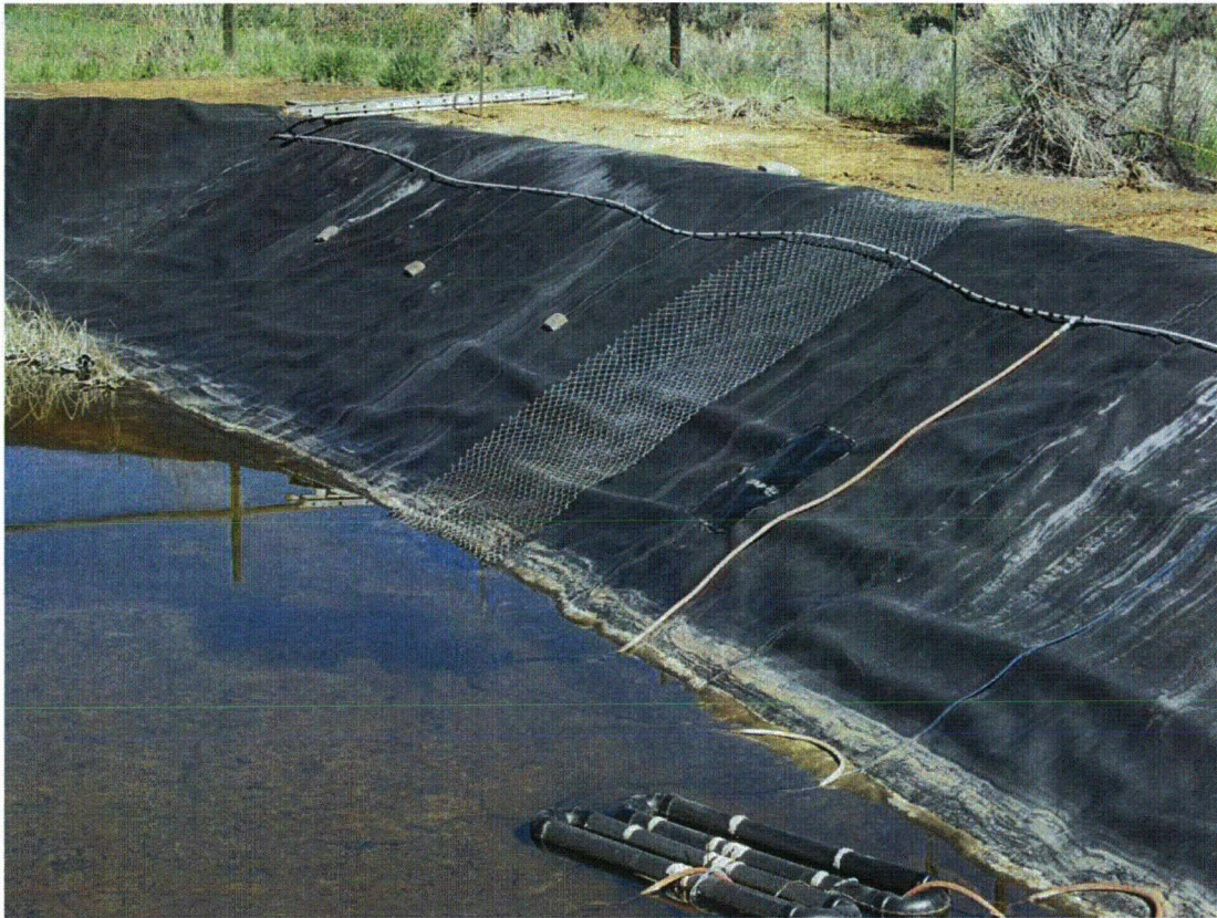
DUD 5/2013. PL-13. Side and liner of evaporation pond.
