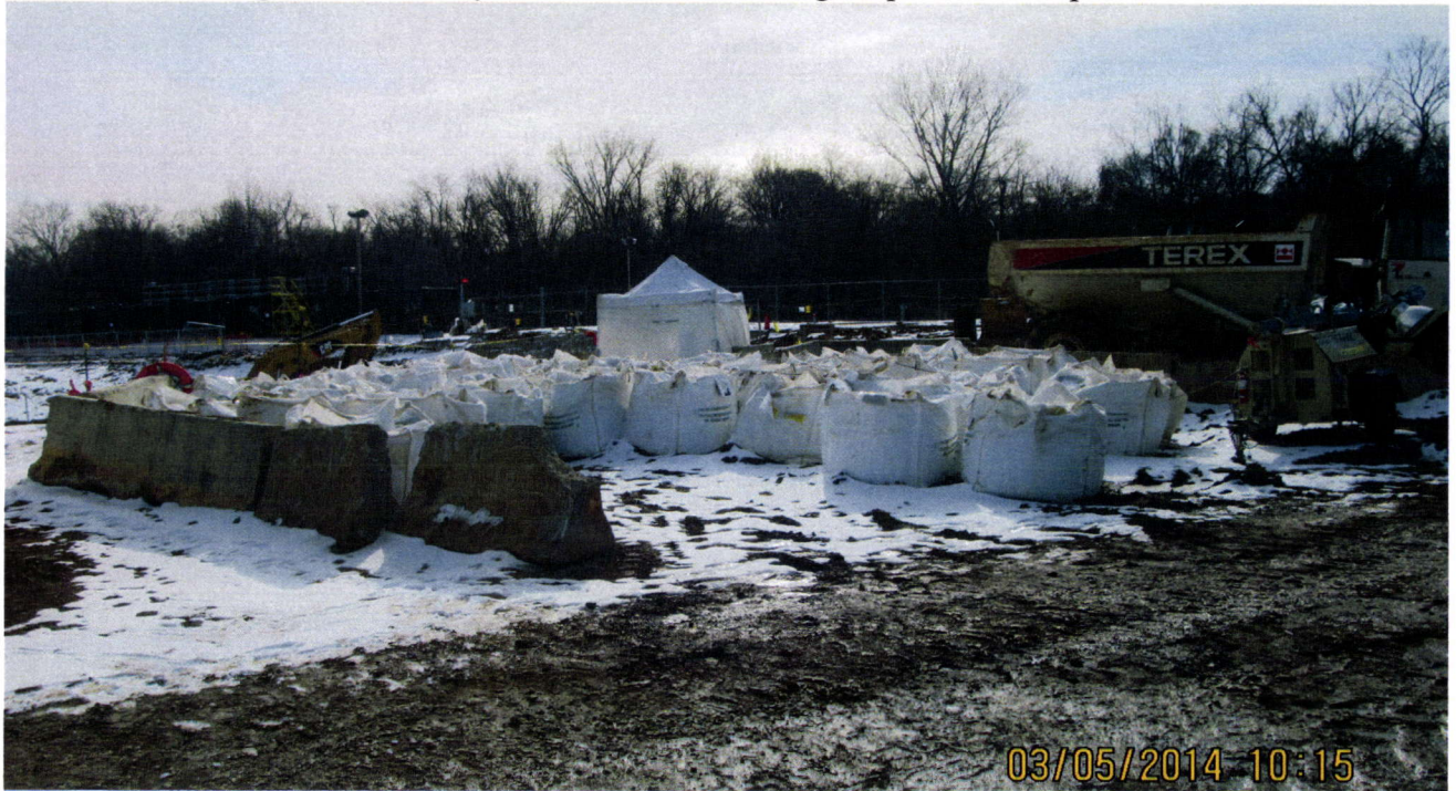
Figure 17. Already Excavated Waste being Prepared for Shipment
